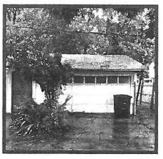
Remove Garage door + replace with hardie backer board that matches the remaining brilding, 2x4x8' boards place at 16' centers to support hardie board, Paint white to match
