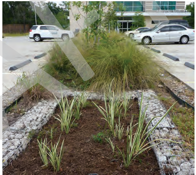
Photo 4.1 (top) and 4.2 (bottom) - The creation of smaller parking areas help to minimize impervious surfaces and create a human-scale environment.
