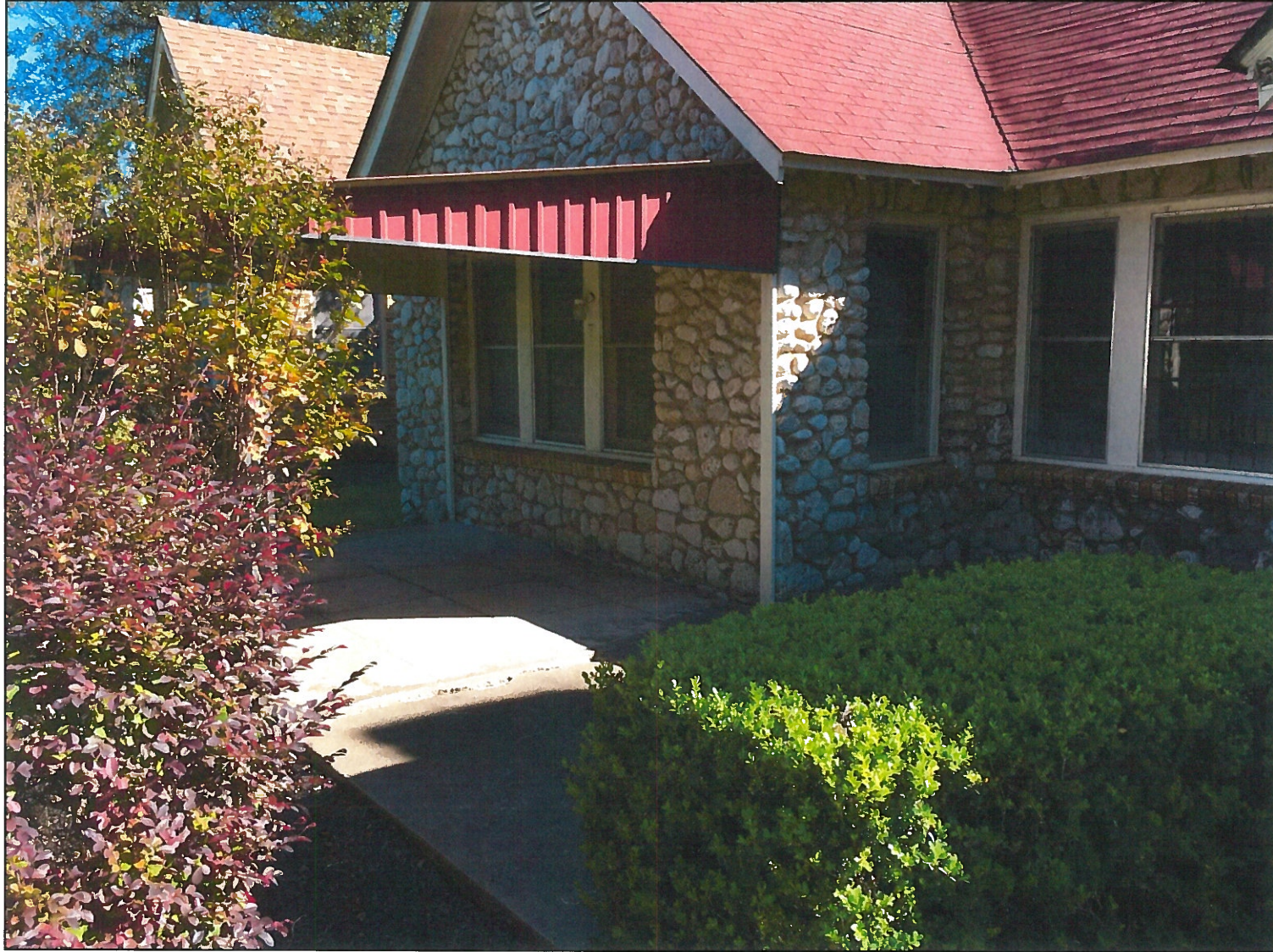
METAL CANOPY & PATIO TO BE REMOVED
