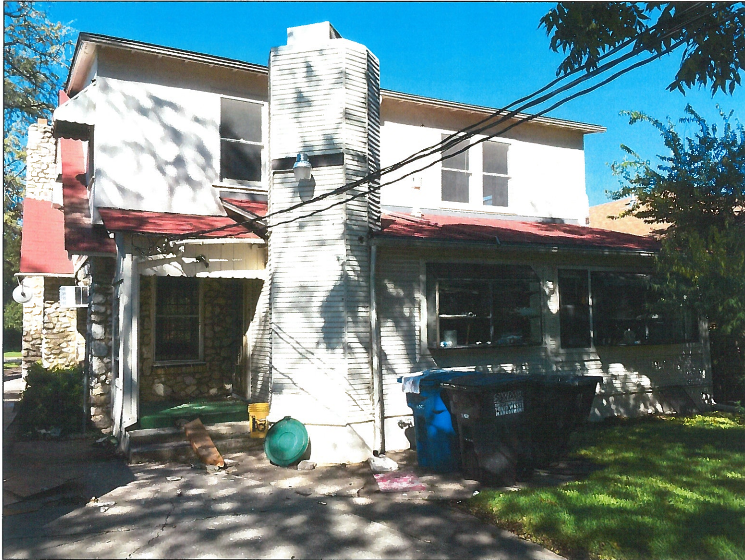
CHIMNEY & BACK PORCH STRUCTURE TO BE REMOVED
