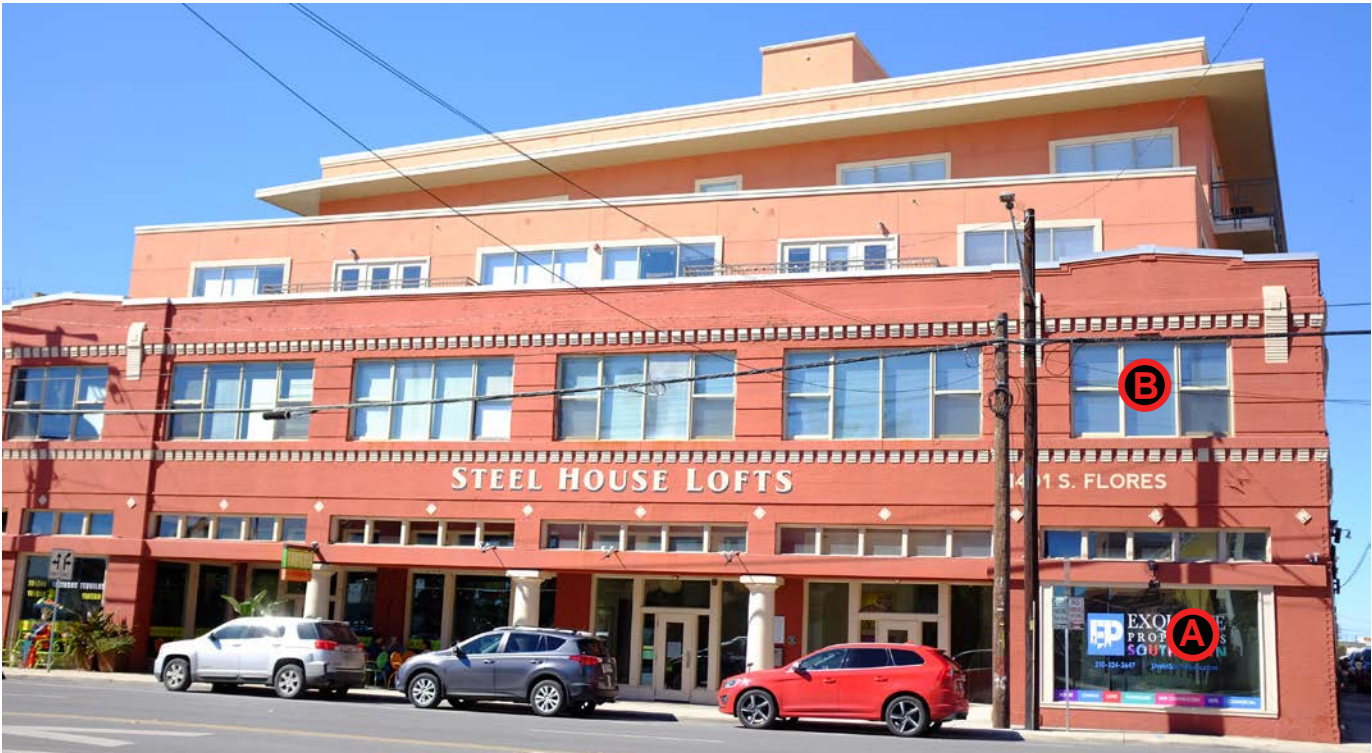
B EXHIBIT B RESTORED WINDOWS WITHIN EXISTING HISTORICAL OPENINGS
