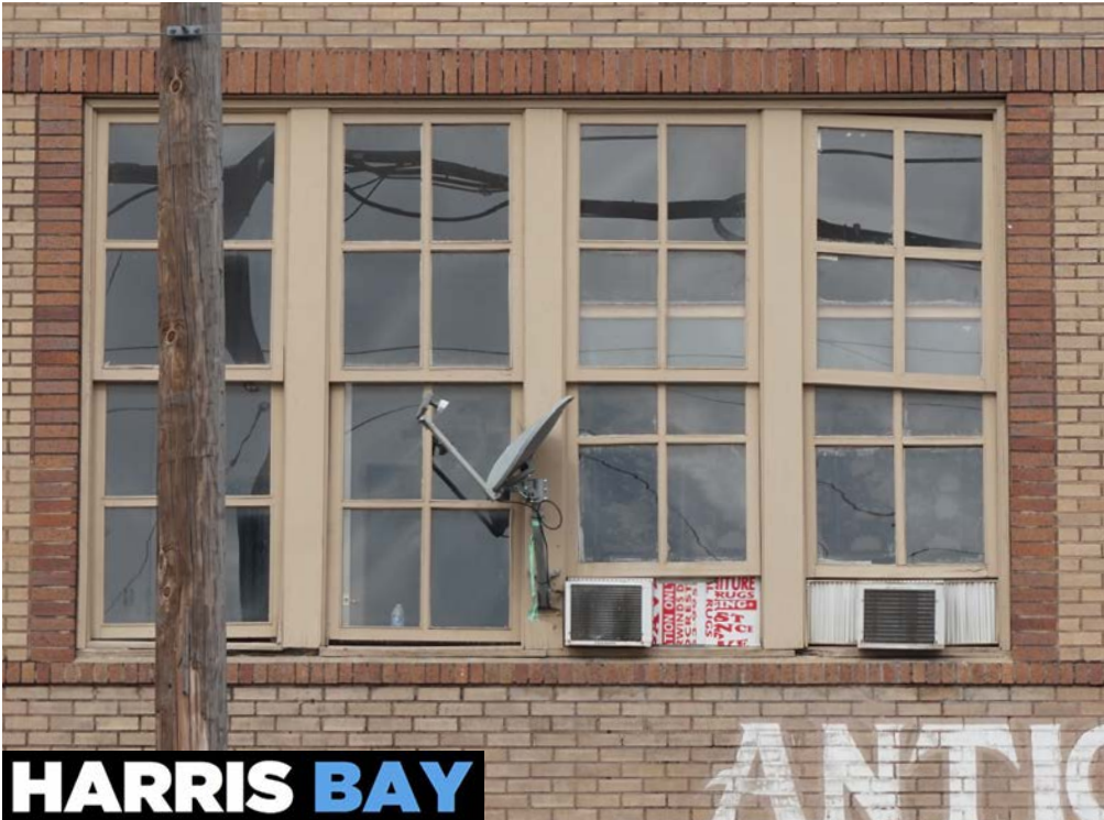
① DETERIORATING SINGLE PANE WOOD FRAMED WINDOWS - TO BE REPLACED (REF. WINDOW SPEC EXHIBIT)
