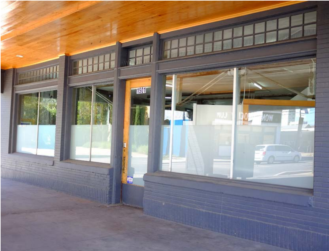
G EXHITBIT G NON-HISTORIC ALUMINUM STOREFRONT W/ FROSTED FILM ON EXISTING STOREFRONT OPENING
