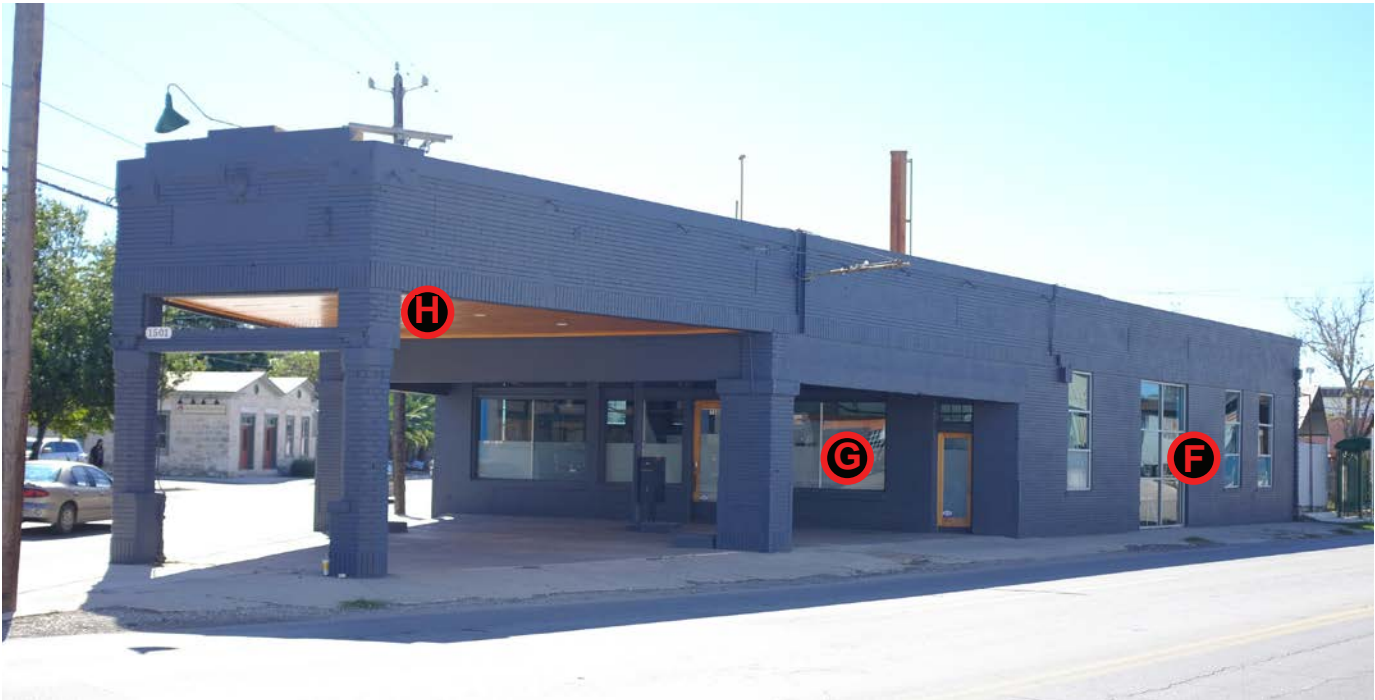
G EXHITBIT G NON-HISTORIC ALUMINUM STOREFRONT W/ FROSTED FILM ON EXISTING STOREFRONT OPENING
