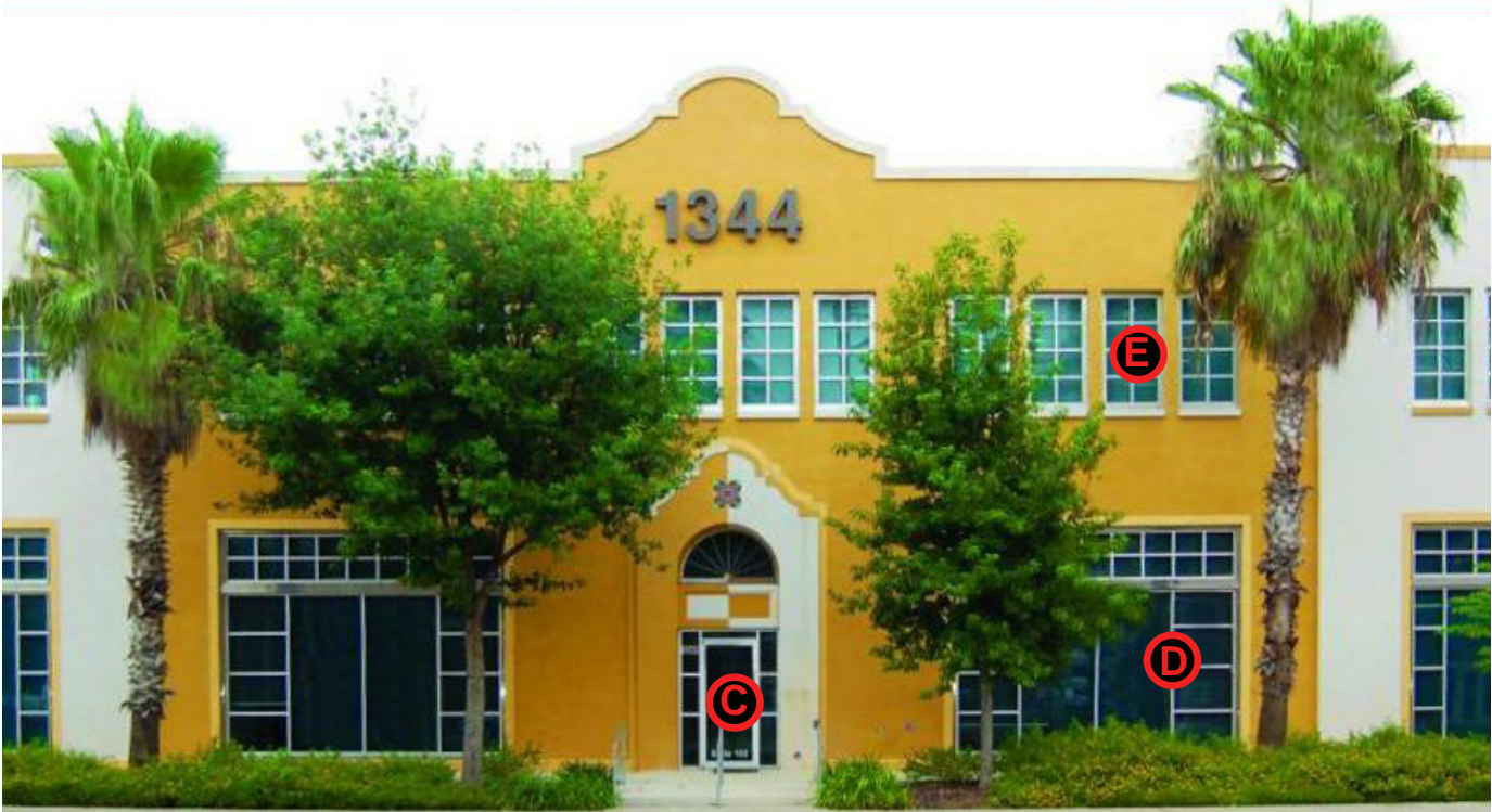
D EXHITBIT D NON-HISTORIC ALUMINUM STOREFRONT W/ TINTED GLASS ON EXISTING OPENING
