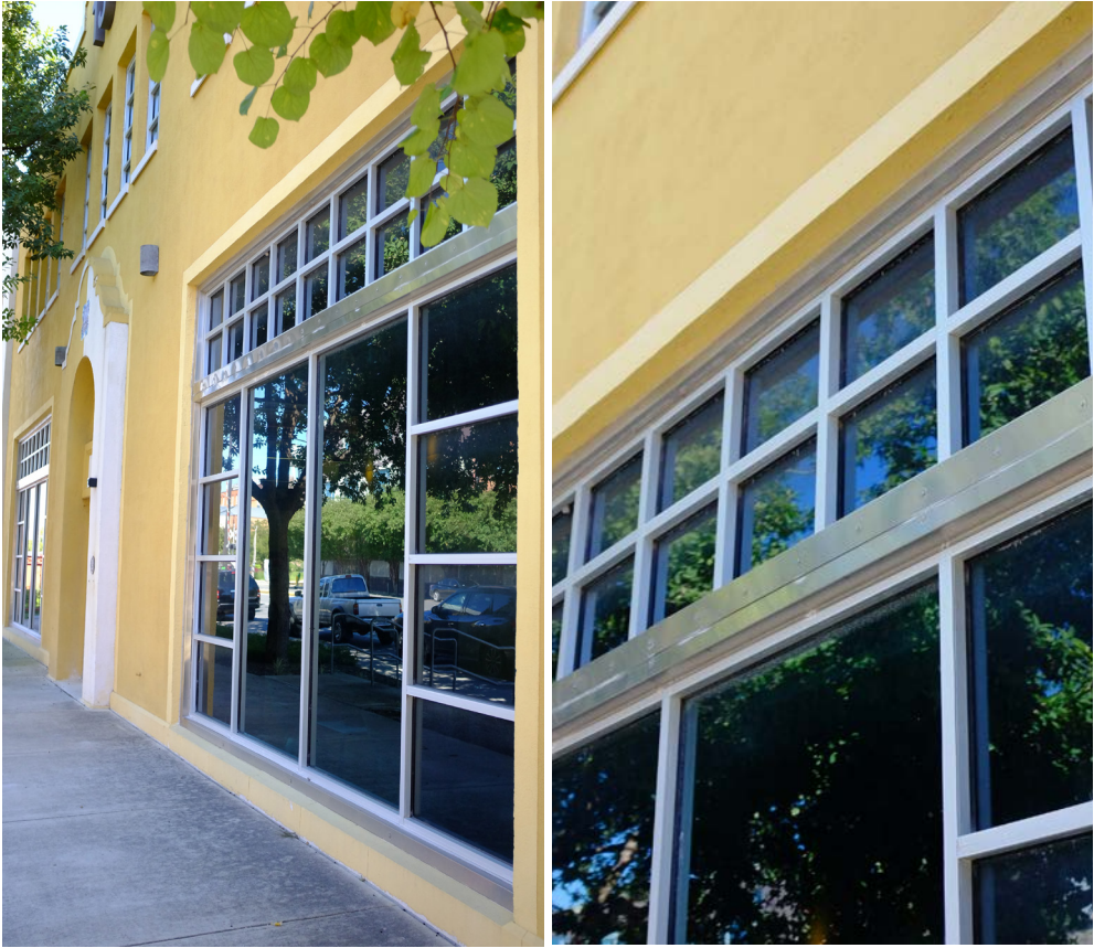
D EXHITBIT D NON-HISTORIC ALUMINUM STOREFRONT W/ TINTED GLASS ON EXISTING OPENING
