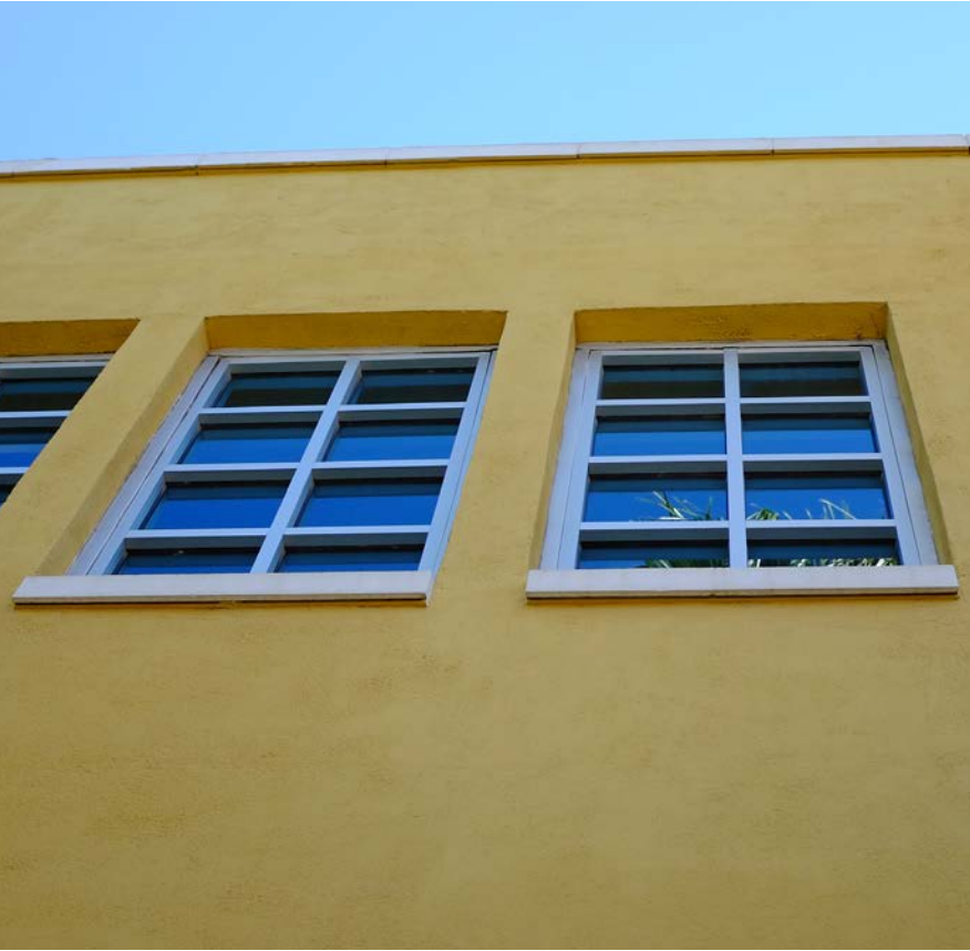
E EXHITBIT E NON-HISTORIC ALUMINUM WINDOWS W/ TINTED GLASS ON EXISTING OPENING
