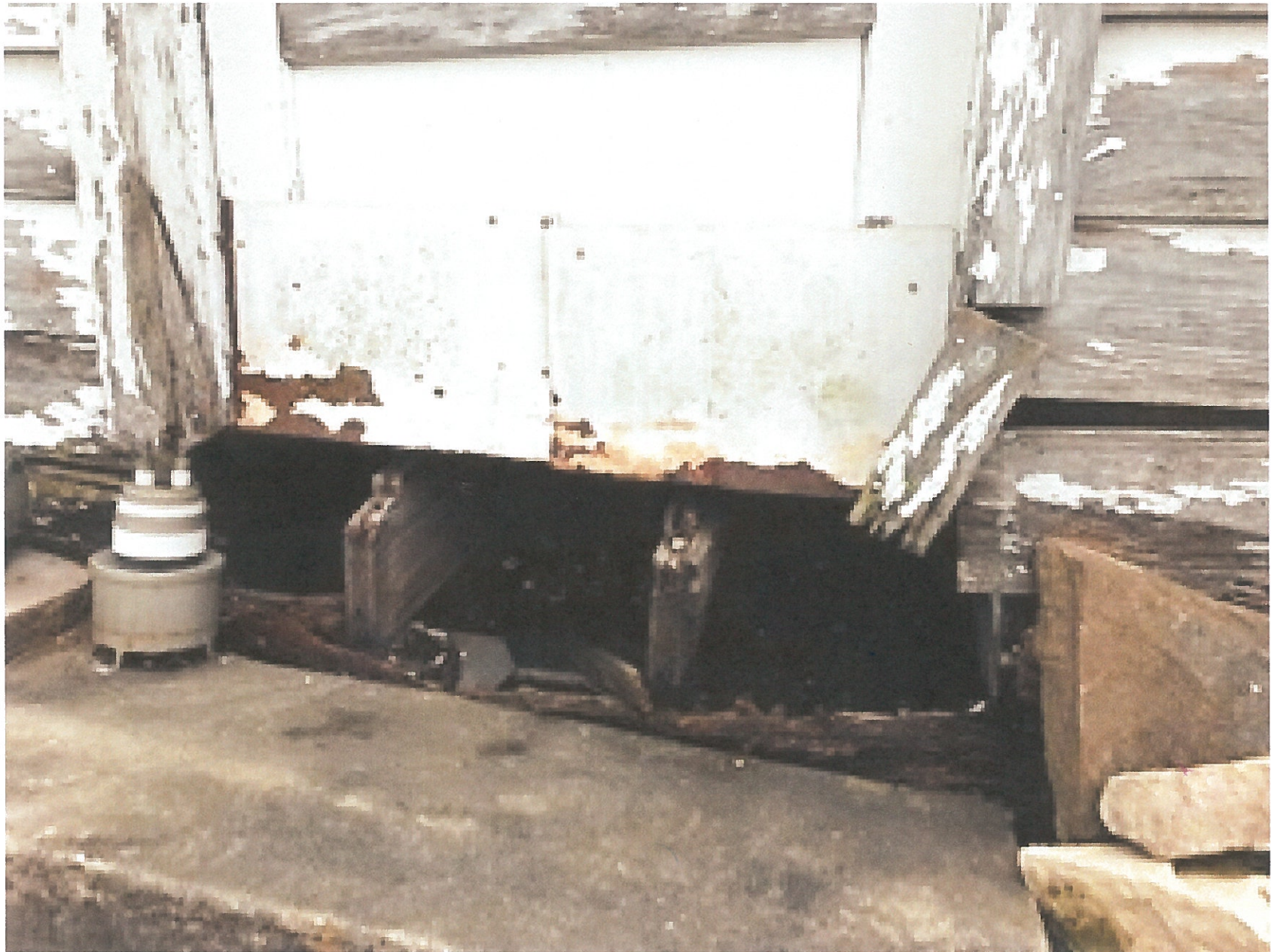
Close up of small building showing rotting floor joists
