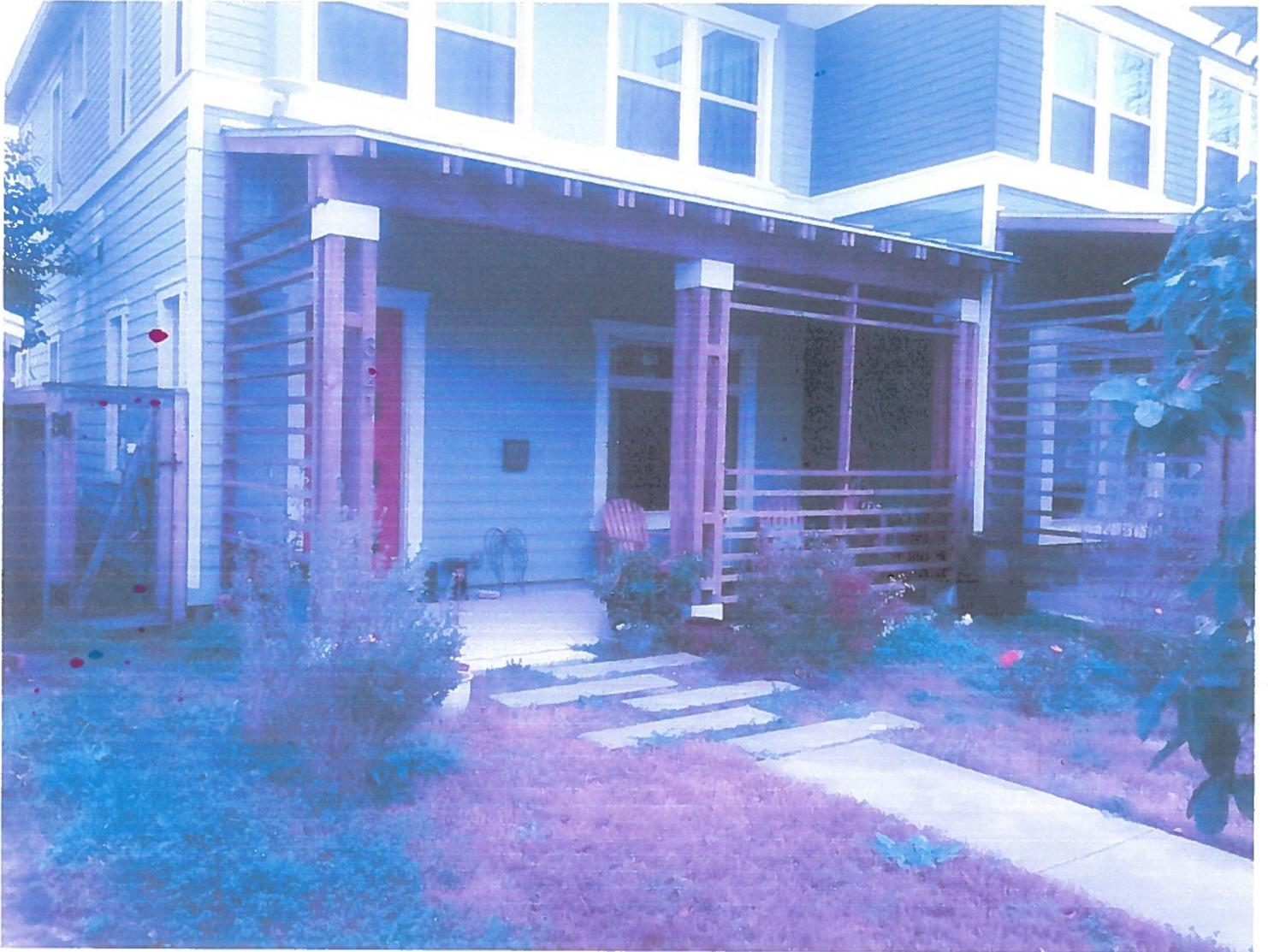
② A CLOSE-UP OF OUR PORCH, CONSTRUCTED OF ROUGH-CUT CEDAR. THE GATE IS 4X4 4 GAUGE HOT WIRE WITH ROUGH-CUT CEDAR FRAME.
