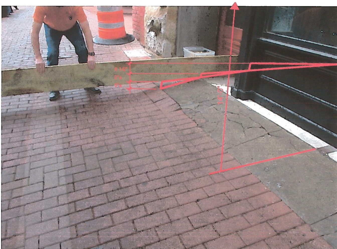
Photo #3: Illustration of the slope of existing sidewalk, entrance does not meet ADA standards
