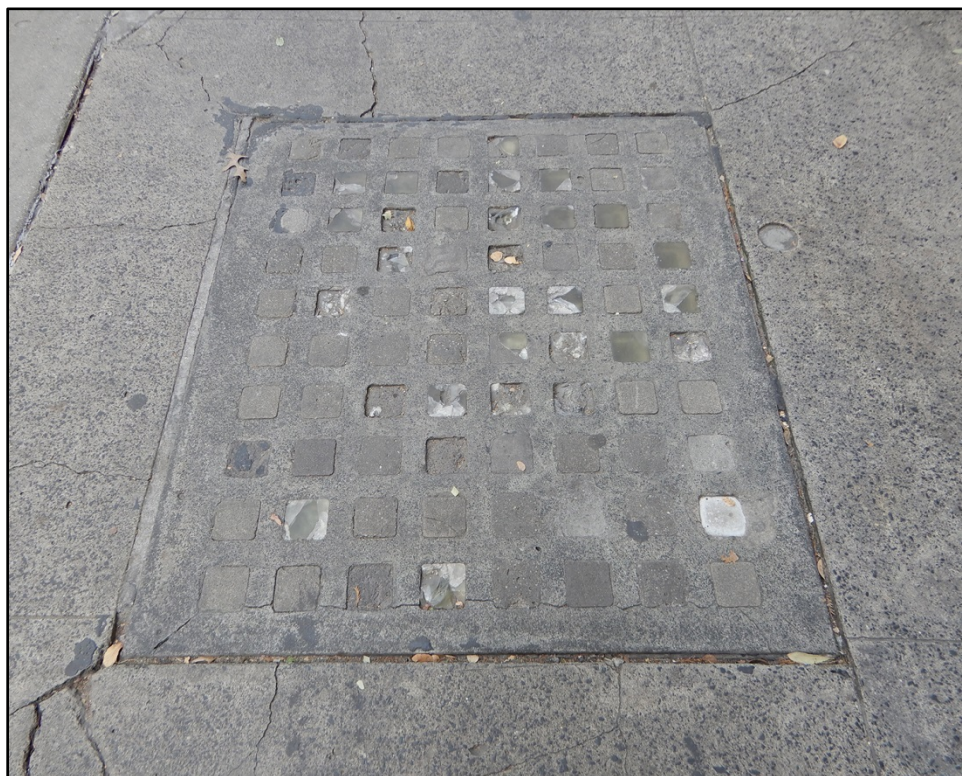
Sidewalk vault light panel 2.
