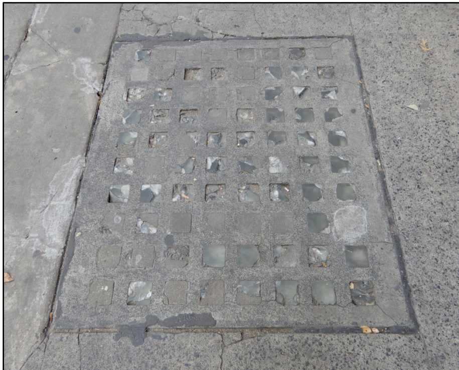
Sidewalk vault light panel 1.
