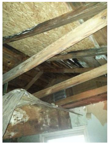
Photo 6 Roof Patch Trusses Infected by Wet Rot and Mold
