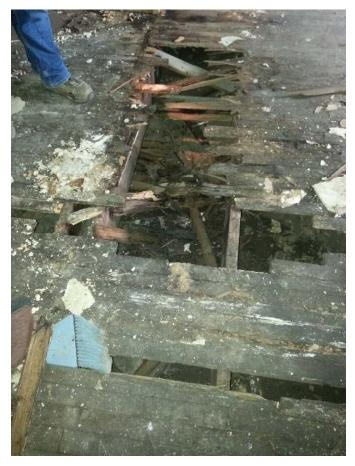
Photo 9 Wood Flooring Damaged by Intruder arrested by SAPD
