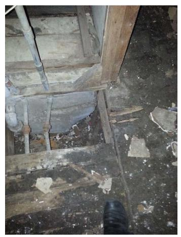
Photo 11 Sheared Steel Water Pipes
