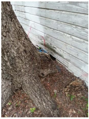
Photo 7 Root Intrusion in the Foundation System
