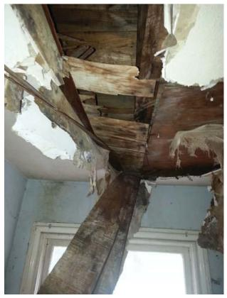
Photo 2 Ceiling Plywood is delaminating and is infested with Wet Rot, Sheetrock is falling
