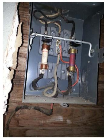
Photo 12 Common Ground and Neutral in Fuse Box. Different Size Fuses on Each Circuit
