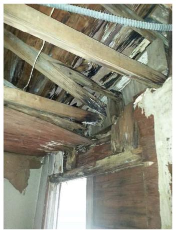
Photo 14 Example of Damaged Roof & Ceiling Framing
