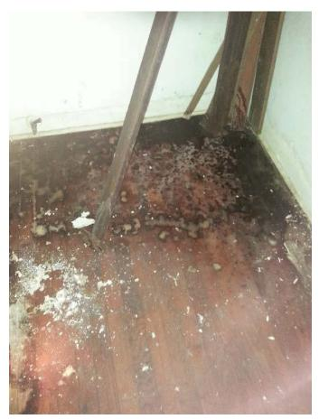
Photo 3 Water damage and Mold on Floors
