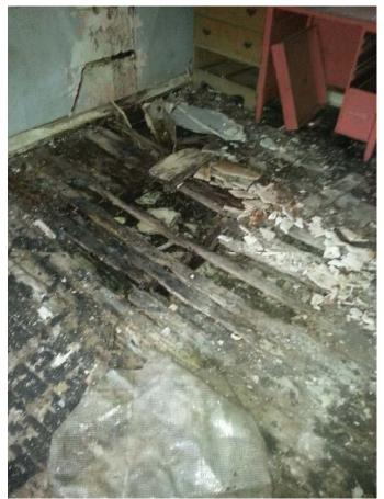
Photo 4 Wood Floor and Wood Floor Joist Deteriorated and/or Missing
