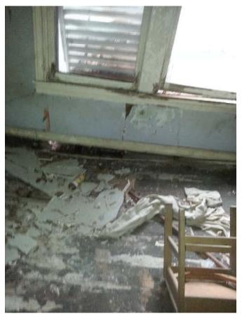
Photo 5 Floor and Floor Joists Fallen Away from the Exterior Wall Floor Base
