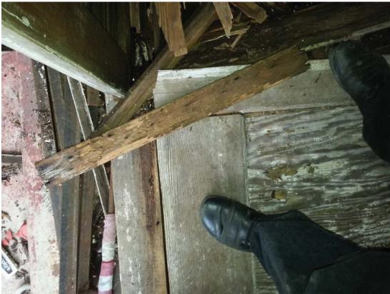
Photo 15 Example of Extensive Termite Damage
