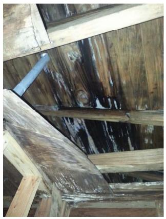
Photo 1 Wet Rot and Mold on Roof Deck
