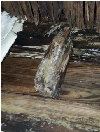
Photo 13 Example of Dry Rot Wet Rot and Mold
