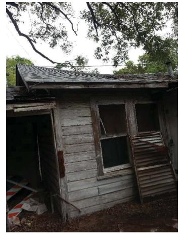
Photo 8 Ridge Beam Broken, Fascia Deteriorated, Composite Roof Deteriorated
