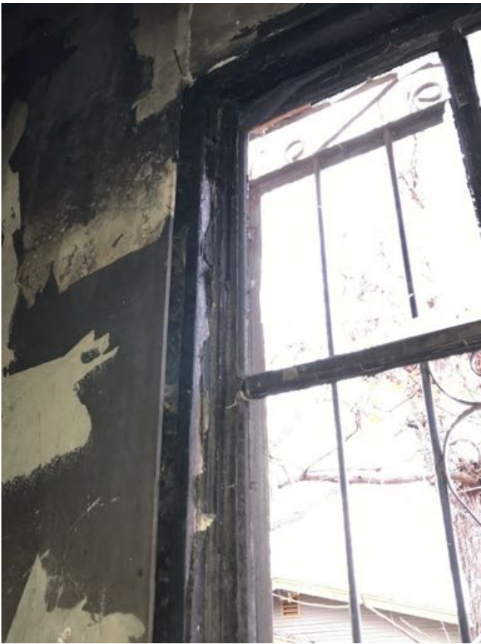
Existing damage to wood windows
