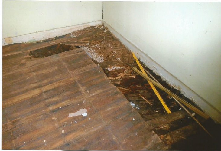
View of damaged wood flooring and deteriorated floor joist and beams.
