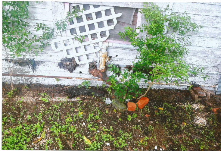
View of the cleanout installed in the sanitary drain line by the South side of the kitchen.
