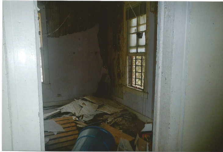
View of damaged wood flooring and wood structure in the bedroom.
