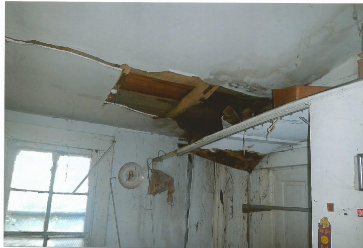
View the damaged ceiling and leaking roof above the breakfast room.
