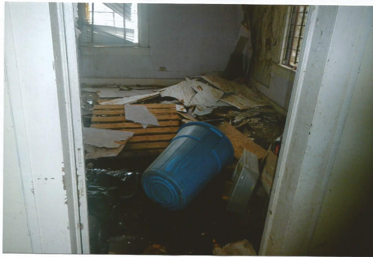
View of damaged wood flooring and wood structure in bedroom.
