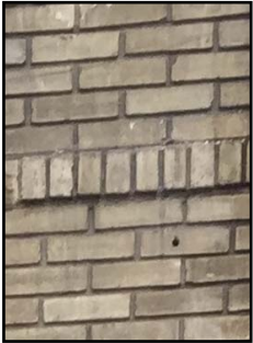
South Building Brick Exisintg Masonry Paint Stripped
