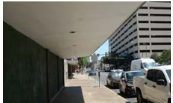
In this instance, recessed downlighting has been installed in a canopy overhanging the right-of-way.
