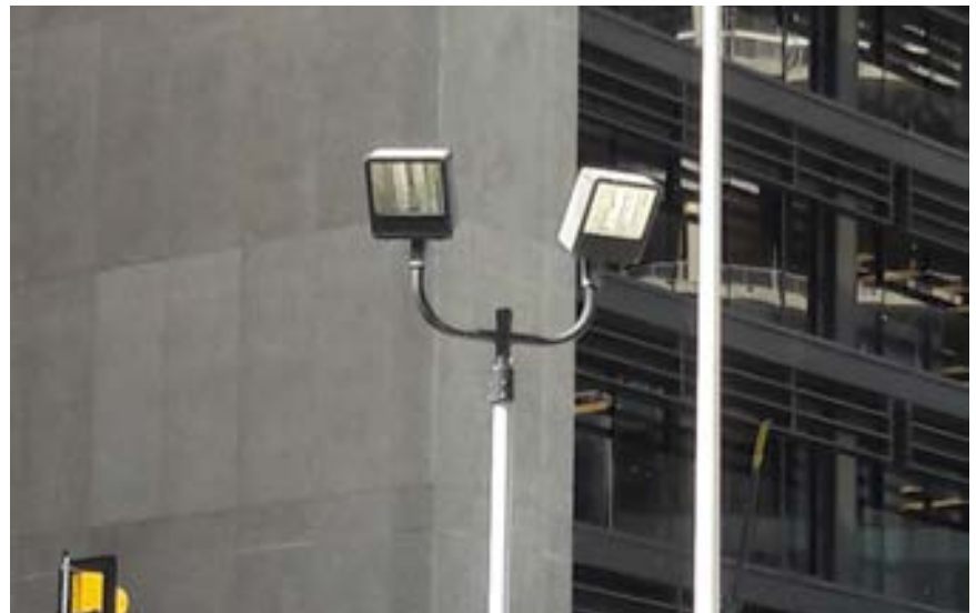
Avoid tilt-up light fixtures focused to produce light above 80 degrees which adversely impact off-site environment. These aiming angles also cause 'skyward' lighting pollution.
