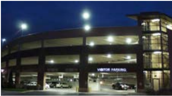
Luminaires with parking structure producing direct glare and nuisance conditions from street level.
