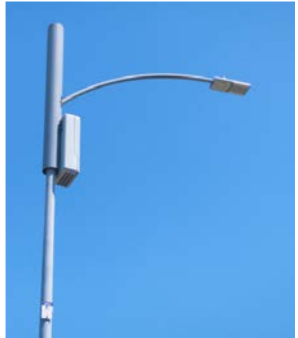
Light pole with antenna and sensor pack
