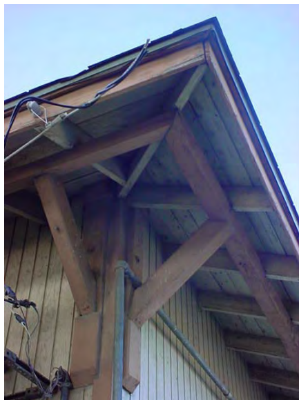
Roof brackets Attachment A
