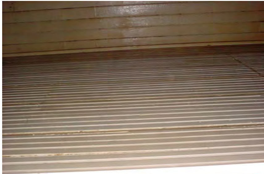
Interior bead board wall and ceiling
