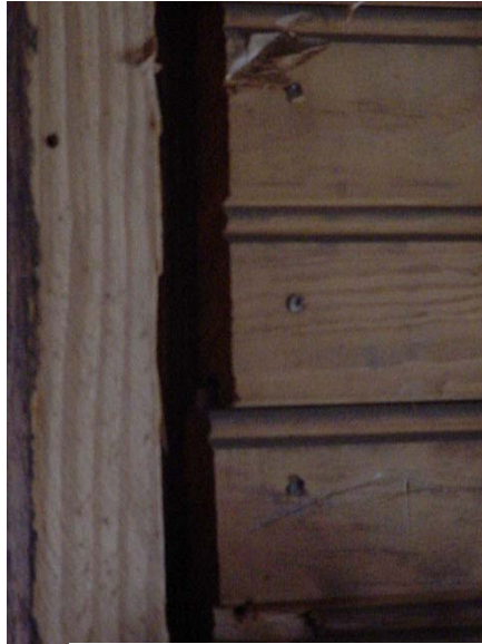
Interior beveled siding Attachment A
