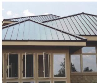
STANDING SEAM METAL ROOF WHERE VISIBLE
