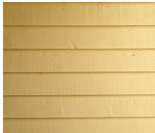
PAINTED FIBER CEMENT LAP SIDING
