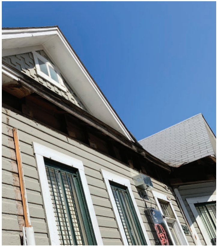
Porch roof and columns damaged and removed
