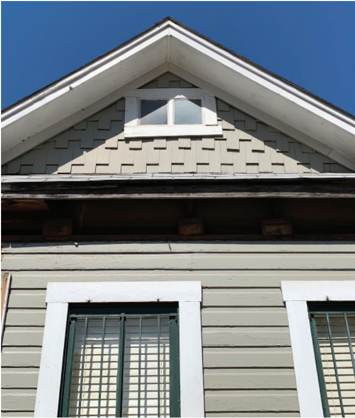
Damaged fascia & soffit
