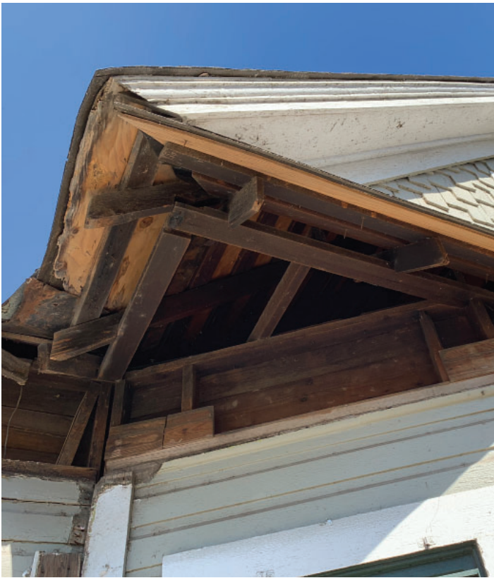
Damaged fascia, soffit, trim, freize boards, decorative running trim
