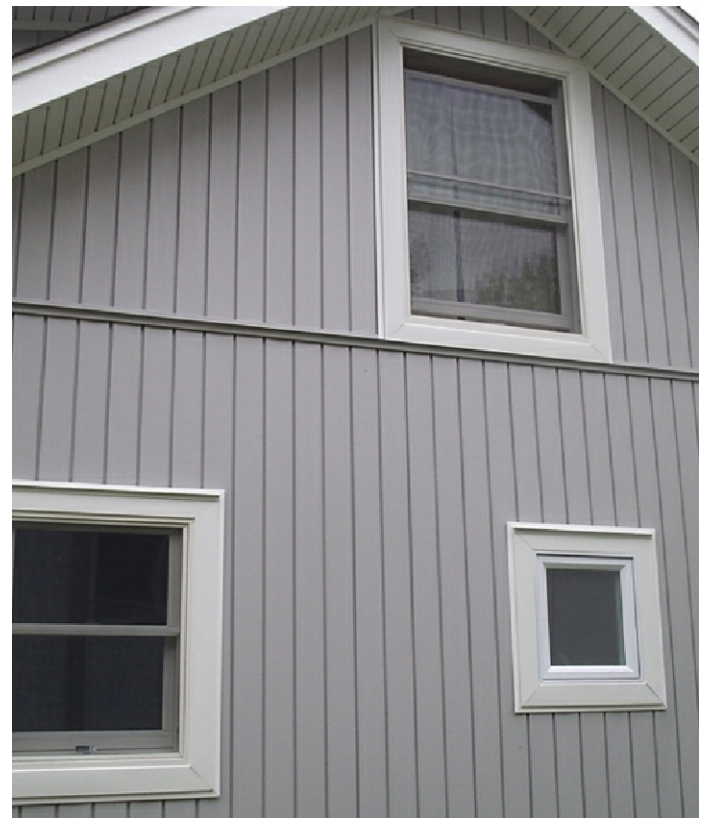
VERTICAL SIDING (T1-11) COLOR: WHITE
