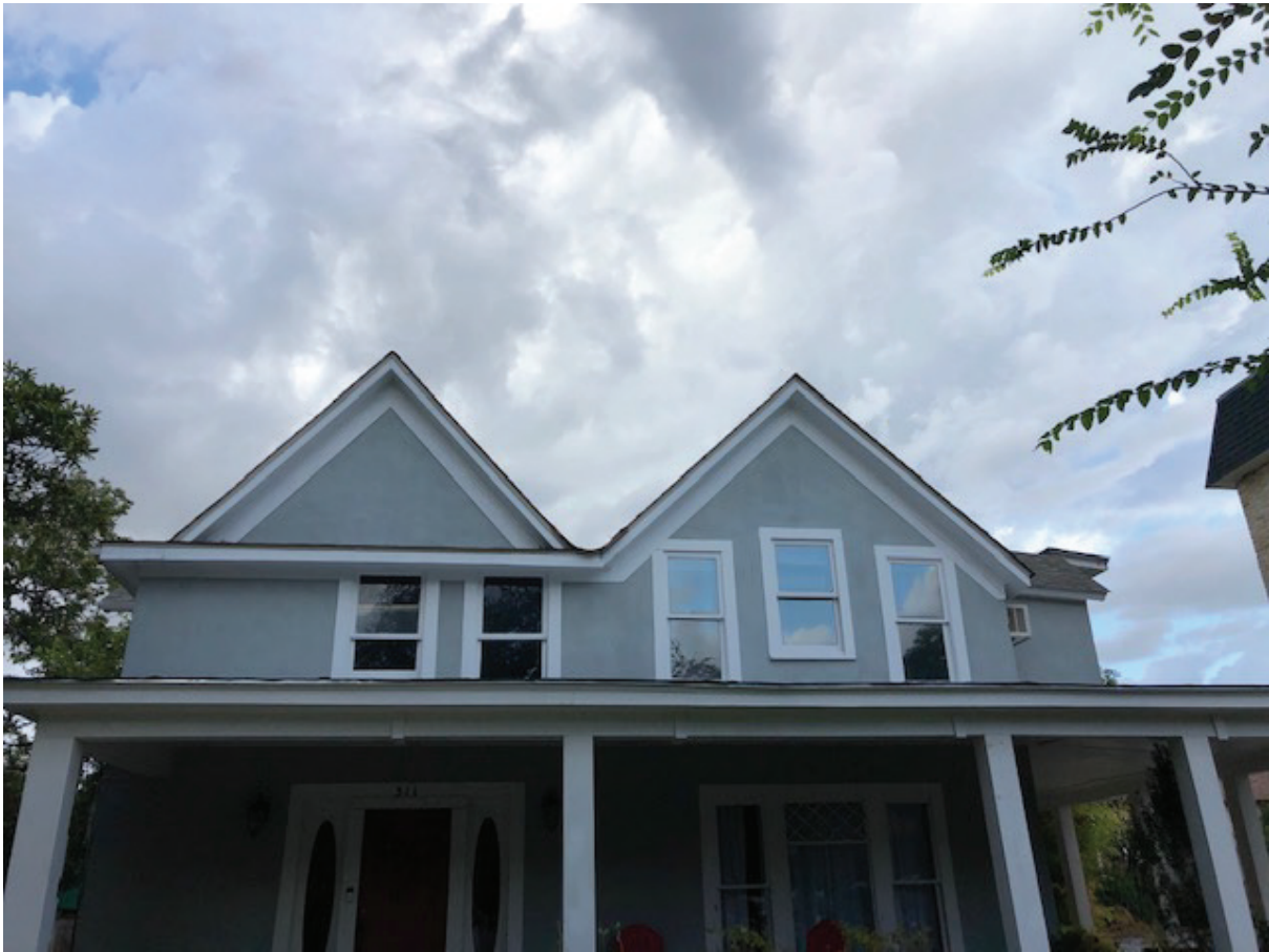
WINDOWS 1 through 5 these will not be replaced
