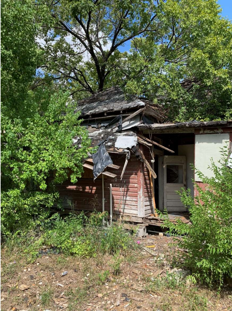
View of back of house with inset and attached porch (not part of original structure)
