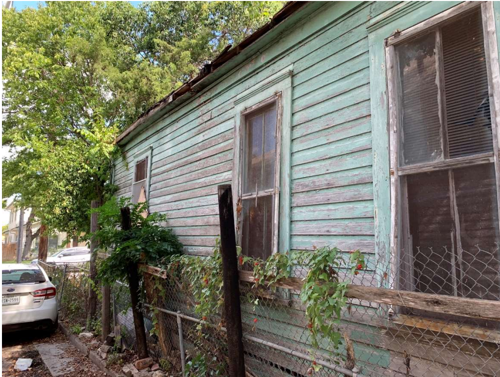
View of right side – windows are aluminum (not original) with wood framed screens
