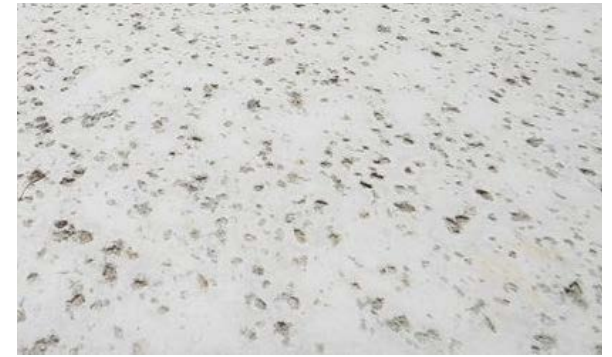
Salt- Finish Concrete Flatwork
