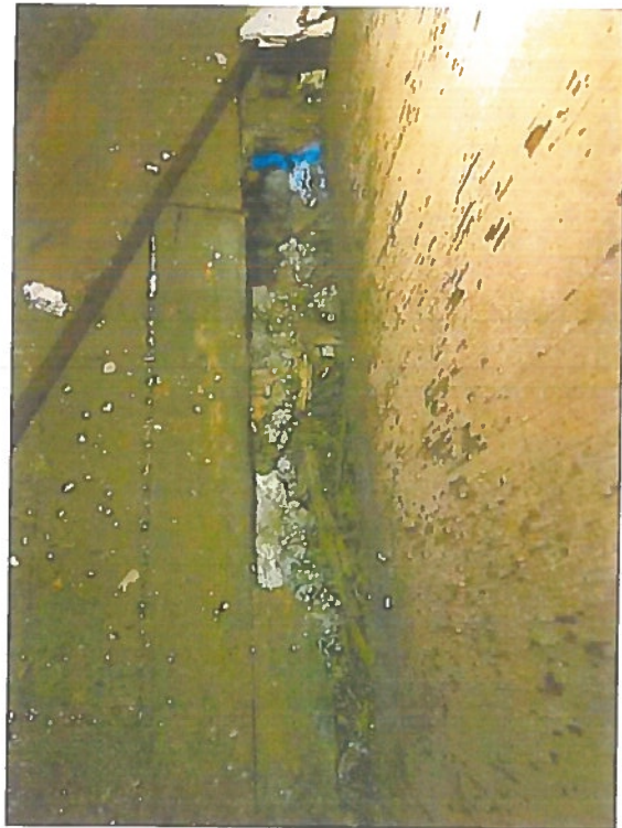
Fig. 5: Floor joists and beam disintegrated at exterior wall, sack concrete used as filler.
