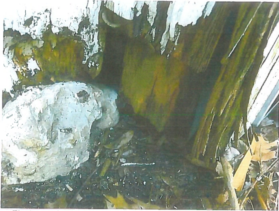
Fig. 3: Exterior post at side door deteriorated. No bottom plate or beam, concrete rubble used to shim gap.
