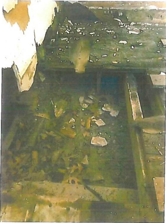
Fig. 6: Interior studs and floor deck deteriorated
