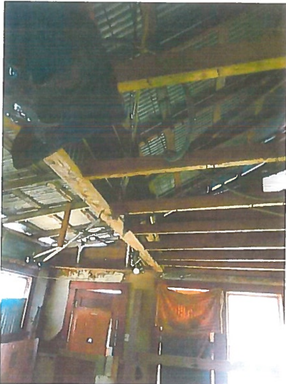
Fig. 4: Rafters and ceiling joists resting on top plate of another missing wall
