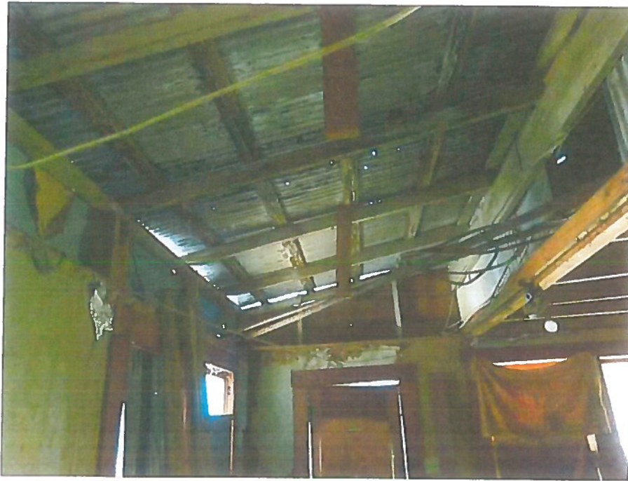
Fig. 1. Interior rafters, pinholes in corrugated roof.
