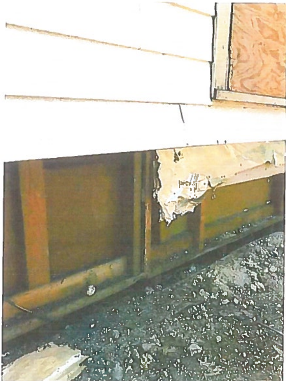
Fig. 9: Exterior joists resting on soil and below grade.
