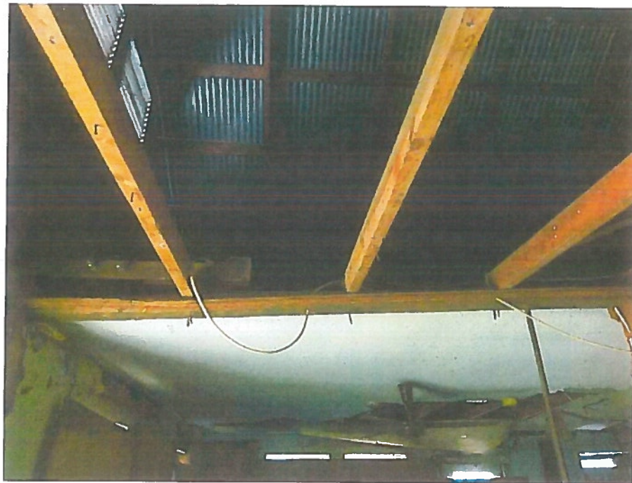
Fig 2: Ceiling joists resting on single top plate, at missing stud wall.
