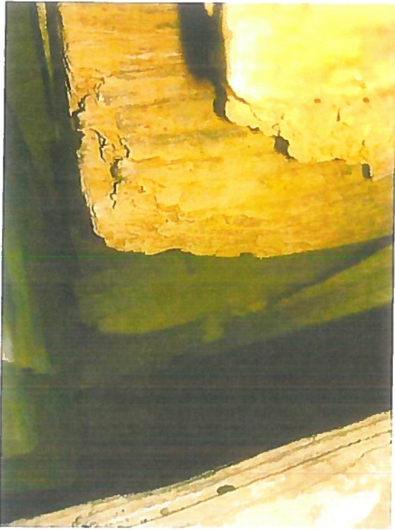
Fig 10: End of floor joist condition, separated from interior wall and beam.
