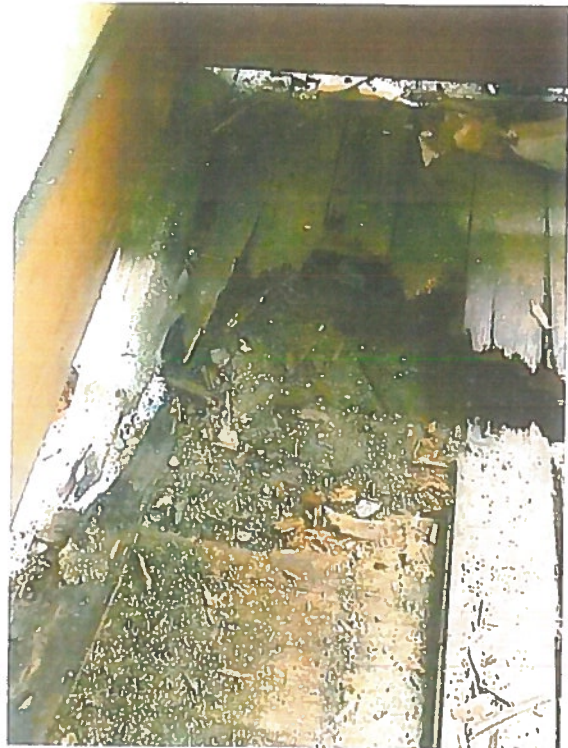
Fig 7: Floor deck disintegrated at exterior corner, no evidence of structural framing support
