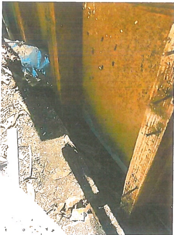
Fig 8: Exterior studs founded on soil below grade.
