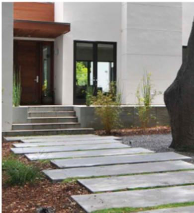
Formed Concrete Walkway
