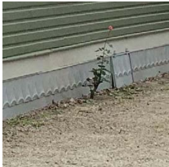
PROPOSED GALVANIZED METAL APRON
