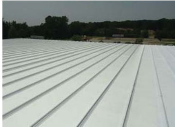
PROPOSED STANDING SEAM METAL ROOF
