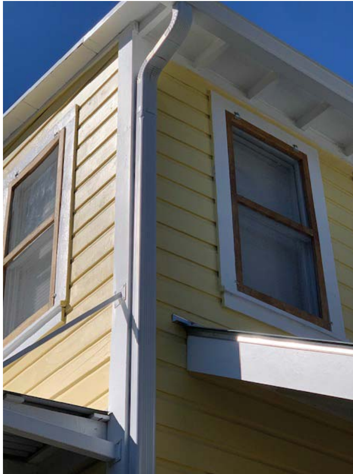
Typical Second Floor Single Hung Windows (South and East Elevations)
