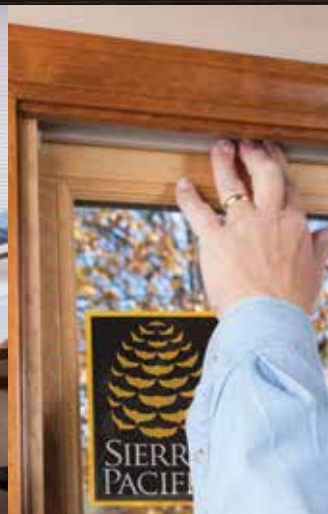
Step 4 Install new head weatherstripping.
