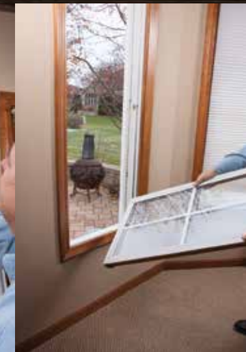
Step 3 Install new sash.
