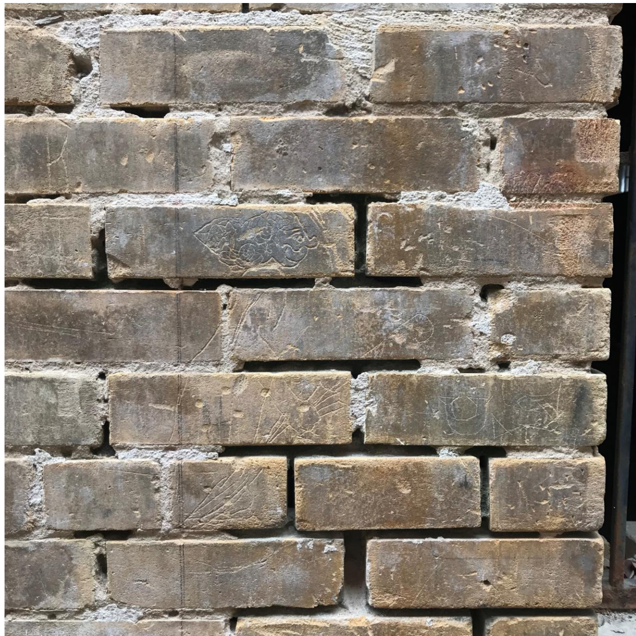
Exterior brick masonry to be repointed and repaired as necessary.
