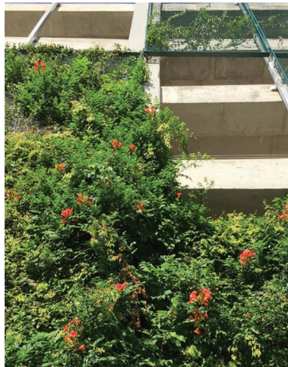
Existing Material Galvanized Trellis Structure
