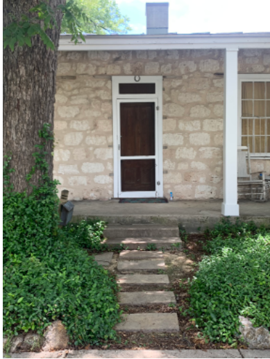
202 Lavaca Stone Pavers
