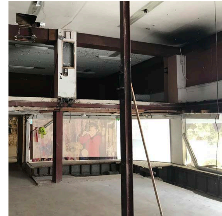
INTERIOR LOOKING AT VESTIBULE AND STOREFRONT
