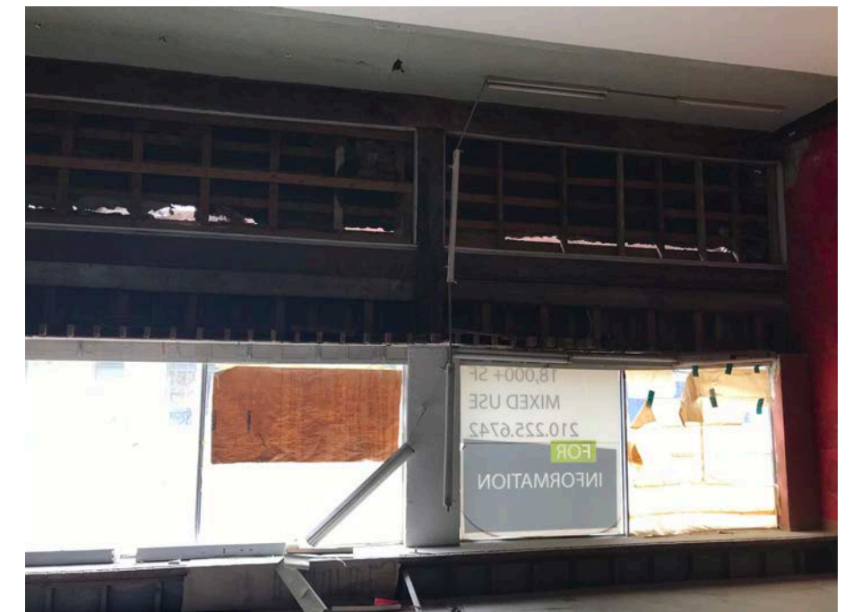
INTERIOR LOOKING AT STOREFRONT AND EXISTING TRANSOM INFILL
