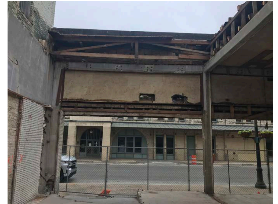
EXTERIOR AT PASEO LOOKING TOWARD COMMERCE ST.
