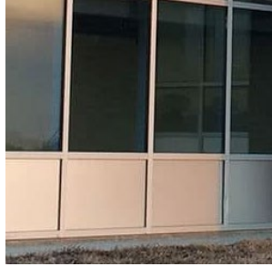
METAL INFILL WITH GLASS (SPANDREL GLAZING WHERE OBSTRUCTED VIEWS ARE REQUIRED)
