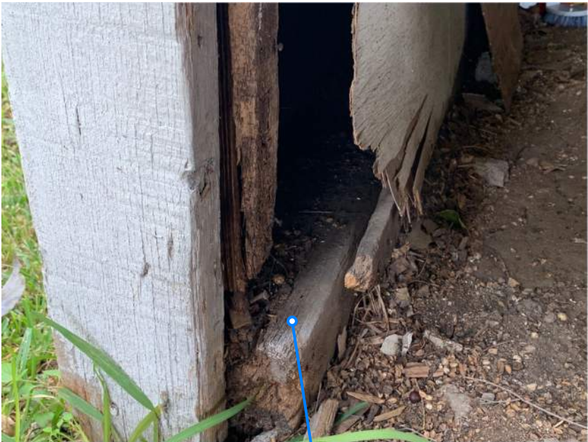
load bearing wall on grade with wood rot and termite damage
