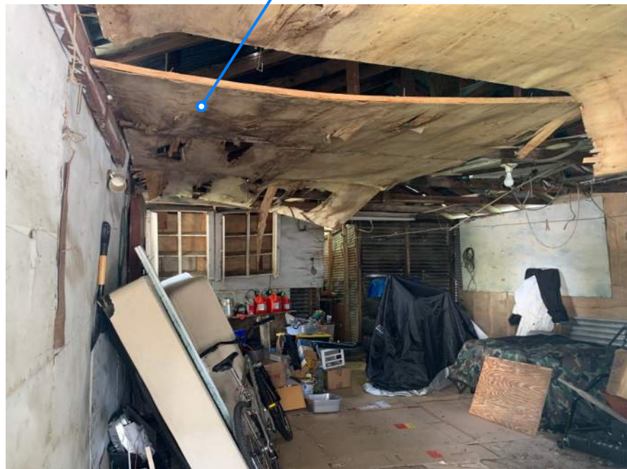
water damaged ceilings + framing
