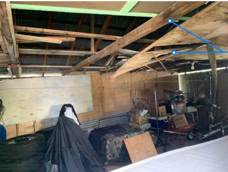
water damage to framing and sheathing
