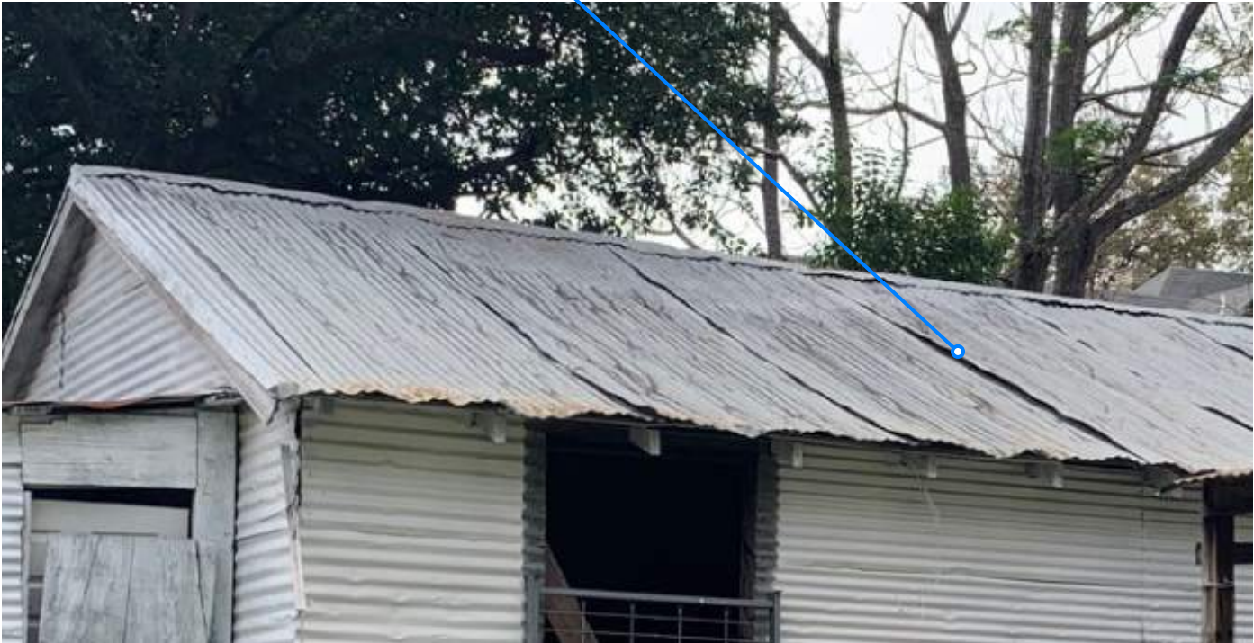
damaged roof panels causing water leaks
