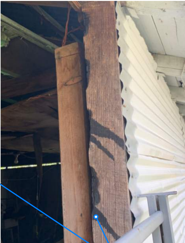
fire damage to wall framing
