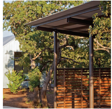
METAL FRAMING W/ CORRUGATED ROOF AT CARPORT
