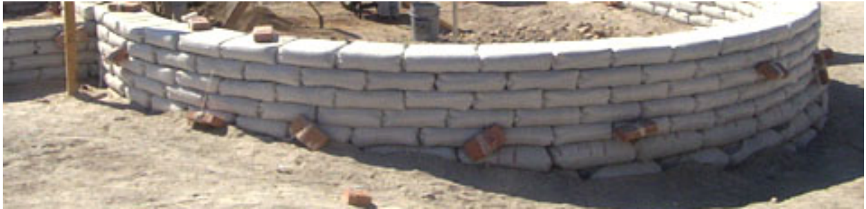
Sample flexible form rammed earth wall structure. To be coated on interior and exterior with a traditional white lime plaster
