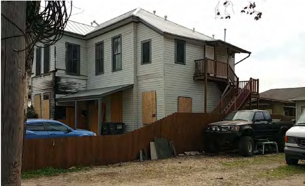
Above and below pictures shows how extensive the wood siding was fire damaged once the aluminum siding was removed.
