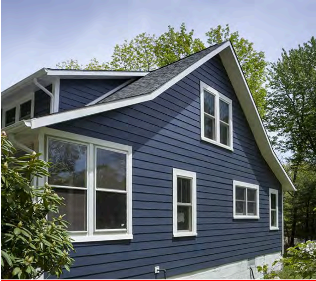
Illustration of composite lap siding
