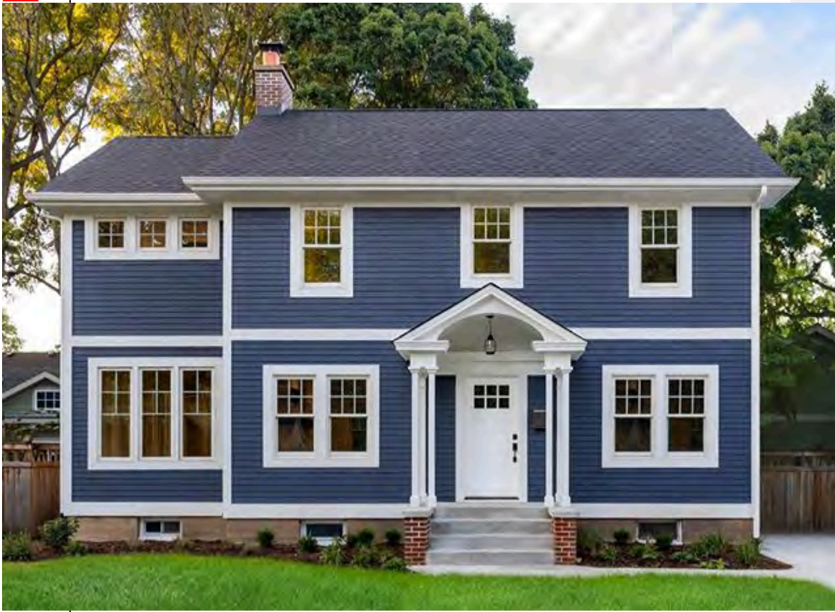
Illustration of composite lap siding
