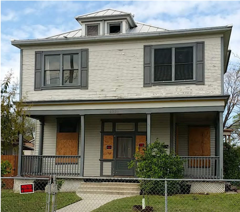
Front of property with waterfall siding, enclosed upper porch, no columns-capitals or bases on porch.
