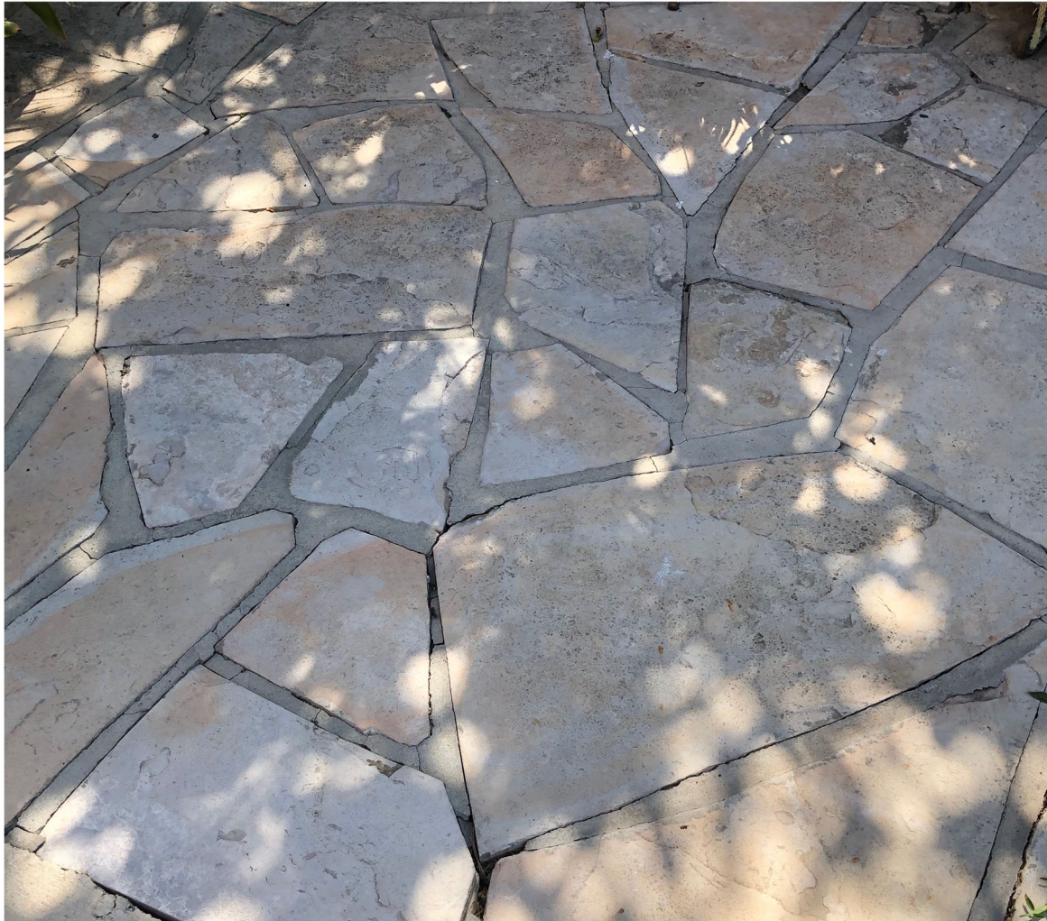
Rosada Flagstone pavers installed in a wet motor mix.
