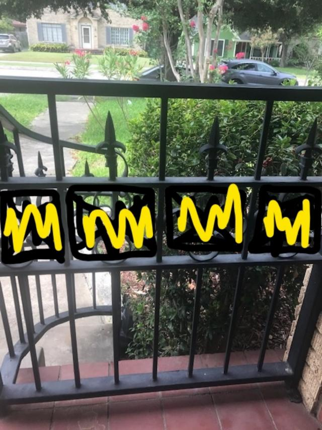
Galvet Ada 311 Post outs cast iron top rail Parters black 3"corner and line POSTS 1/2" solid pickers 1 × 1" solid sai Cast iron finials + post caps 1/2" solid pickets 1"x 2" solid bar rail 1"x 1" solid par vail Concrete 3 deep 3" corner + line post 1/4" thick
