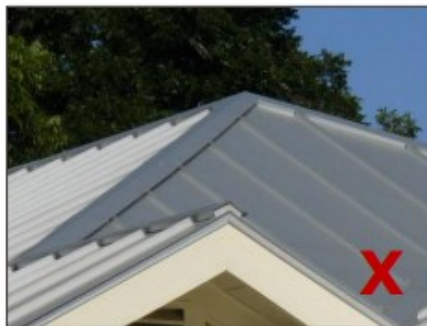
Do not use ridge caps with vents (left) or end caps (right).
