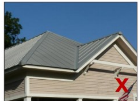
Do not use ridge caps with vents (left) or end caps (right).
