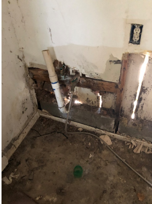
3. Typical sole plate conditions.
