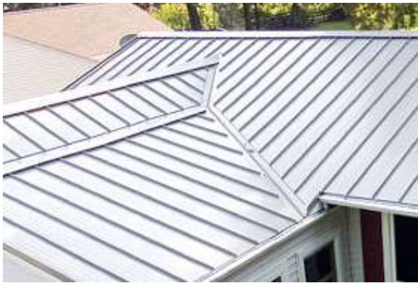
STANDING SEAM METAL ROOF
