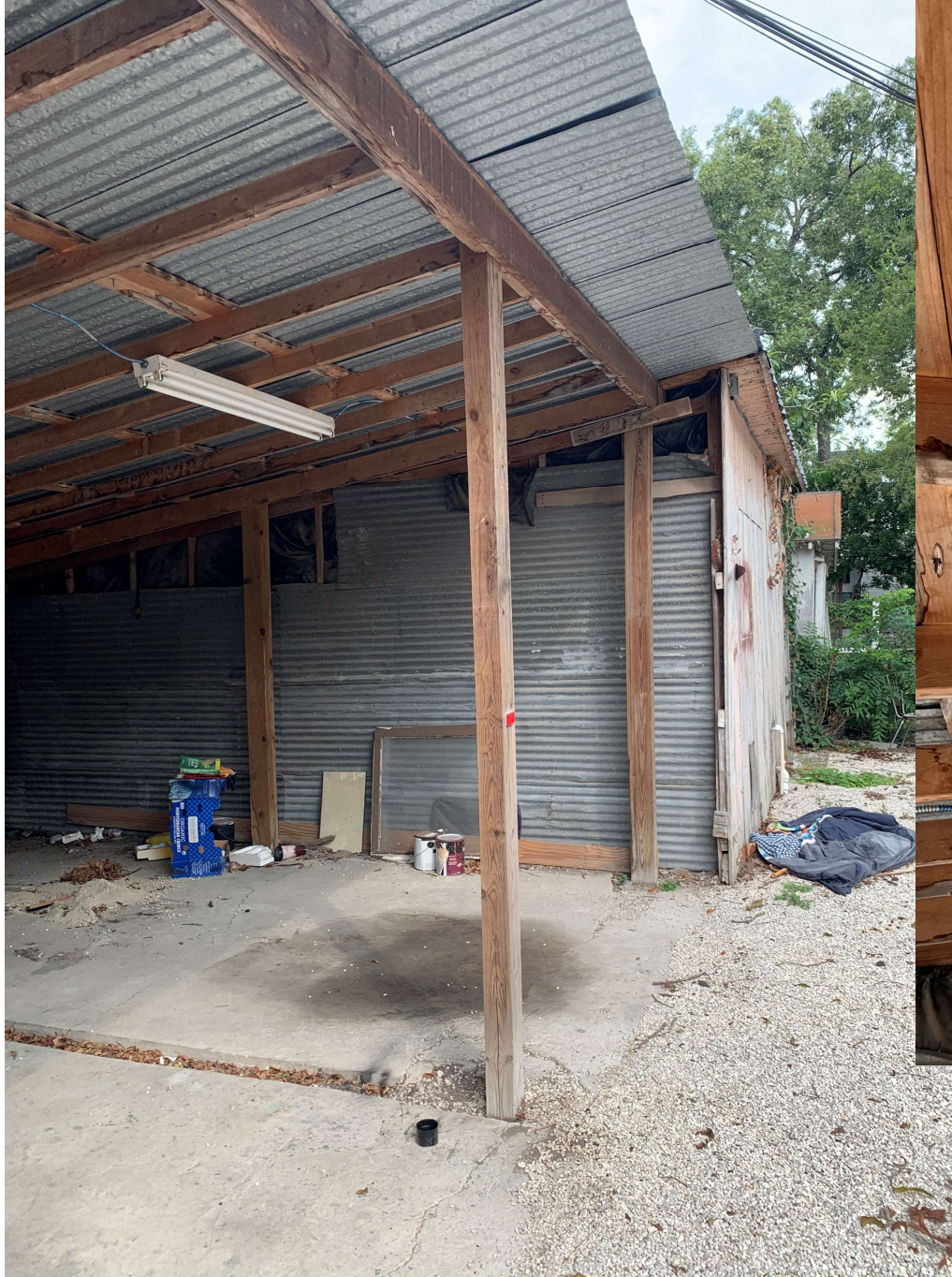
Existing Accessory Structure Dimensional/Treated Lumber, Corrugated metal, non-historic materials. Structure partially built directly on ground.
