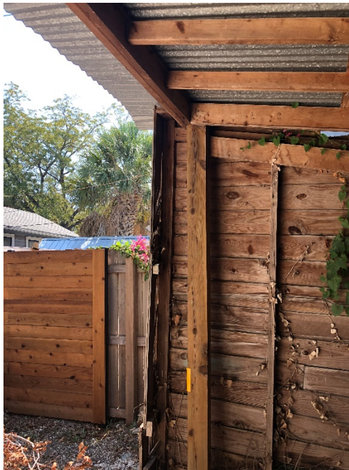
2. View of header and post lack anchorage to wind uplift.
