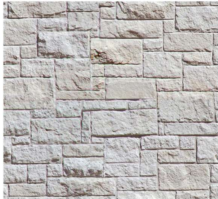
STONE VENEER (MATERIAL): COBRASTONE WHITE LIMESTONE REGULAR CHOP
