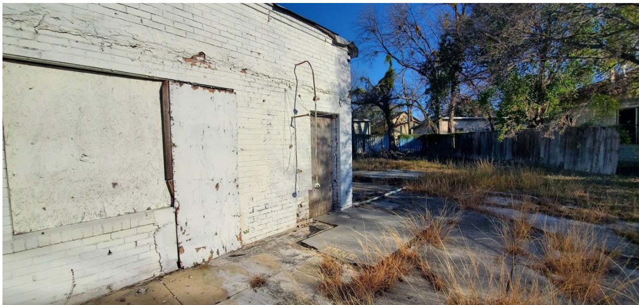
Tiled concrete slab on southeast side
