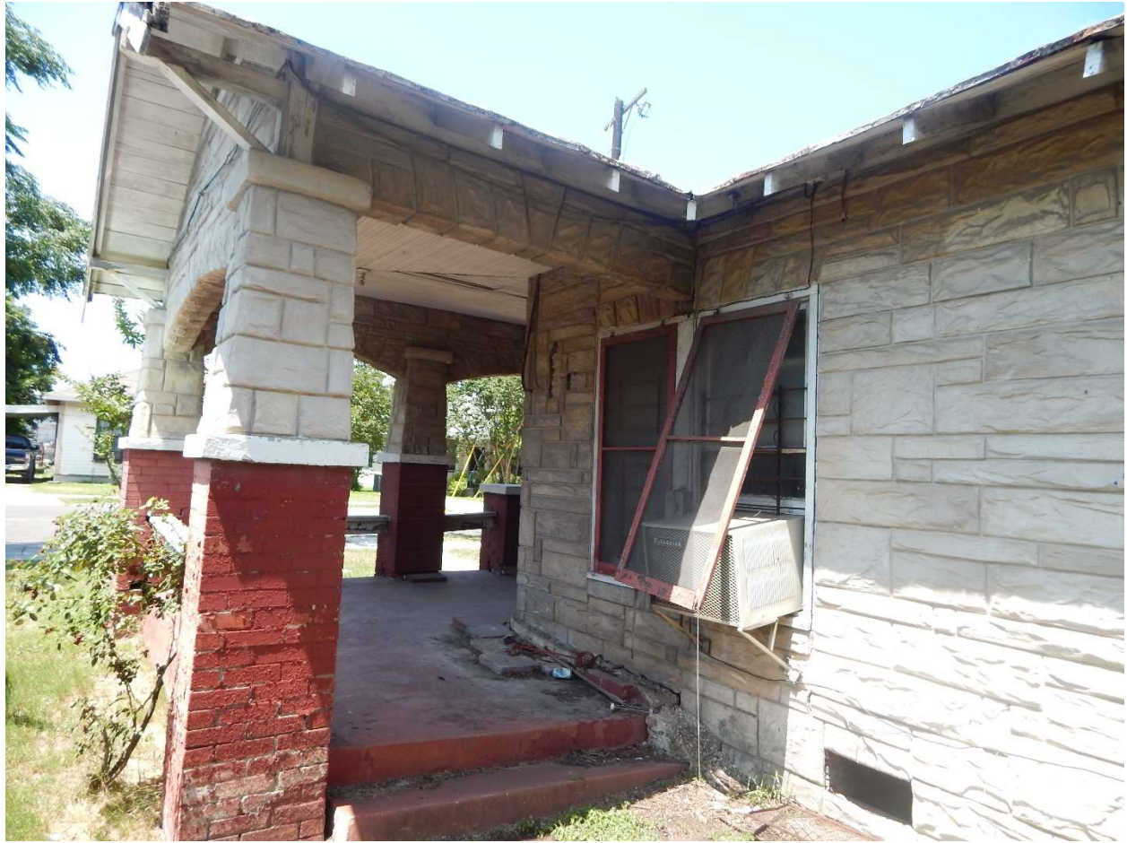
Figure 5 – Right exterior of sinking porch.
