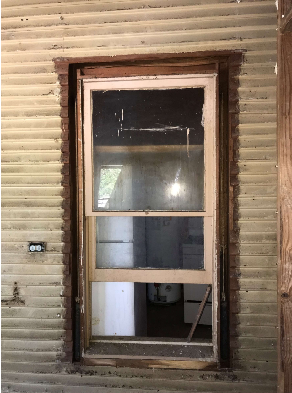
Figure 18– interior original window (hidden) between kitchen and addition added in 1930s or 1940s
