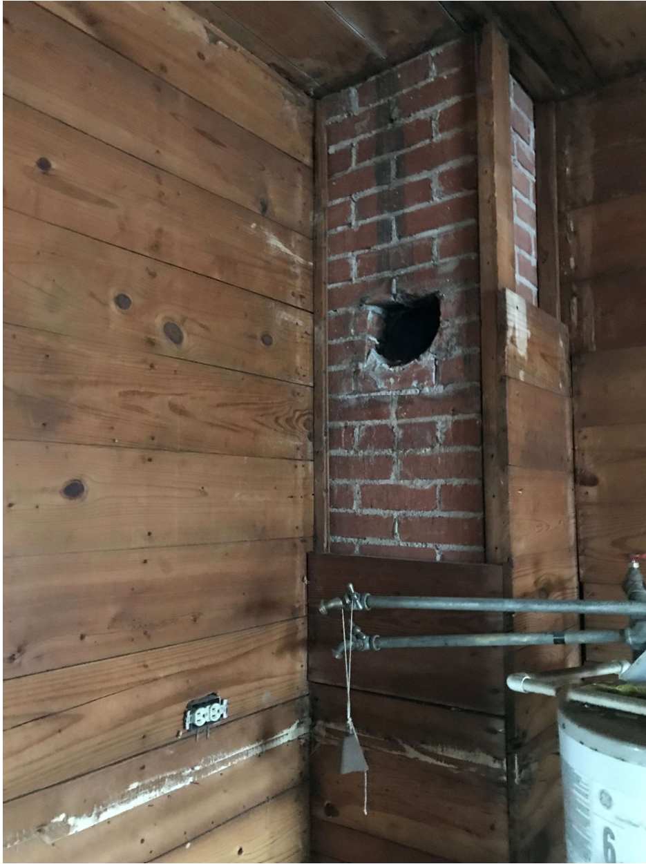
Figure 13– interior kitchen chimney with wash connections/waterheater
