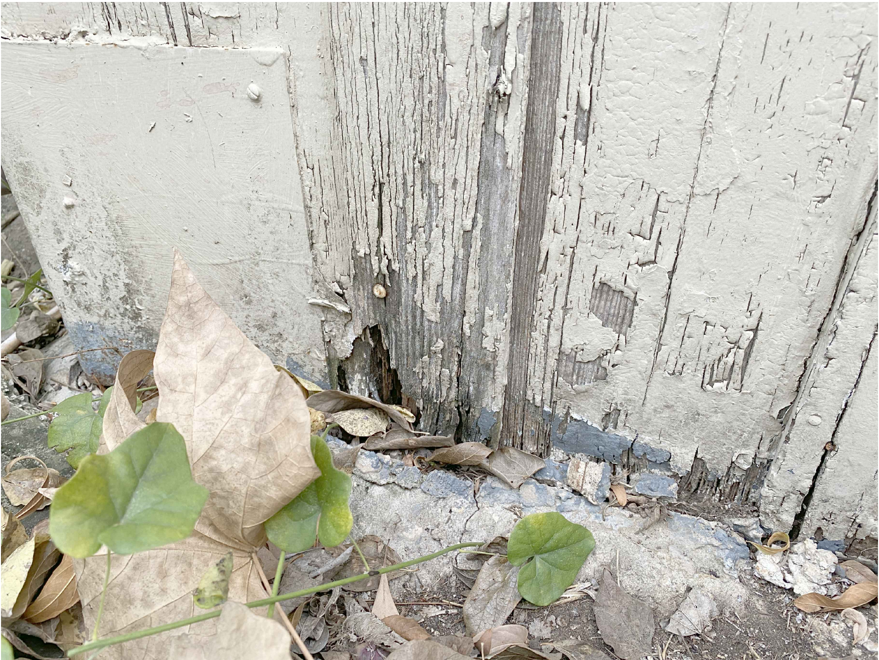
TYPICAL DETERIORATION AT BASE
