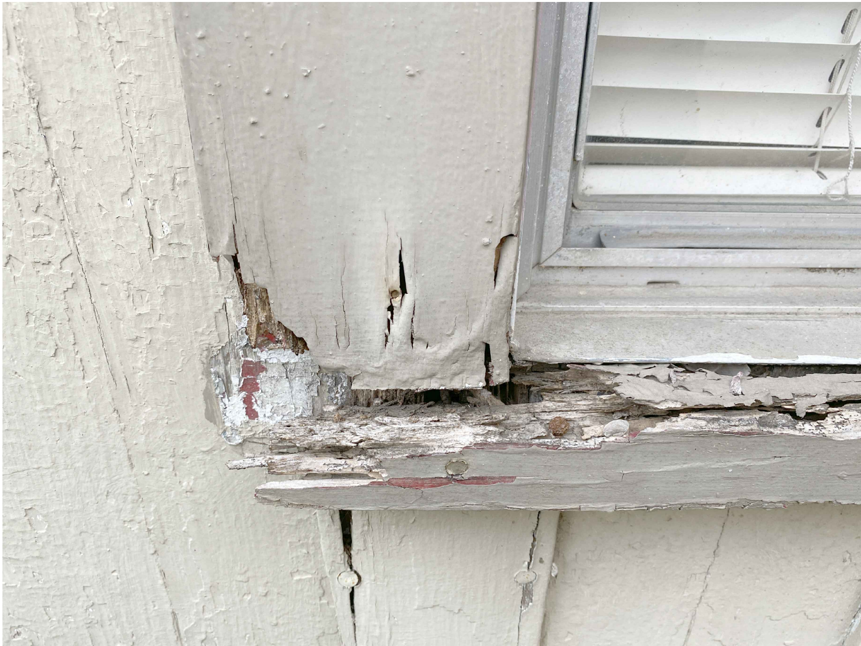
TYPICAL DETERIORATION AT WINDOWS
