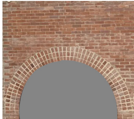
EXISTING BRICK: REMOVE ALL PAINT, CLEAN, REPOINT GROUT AND SEAL CLEAR.
