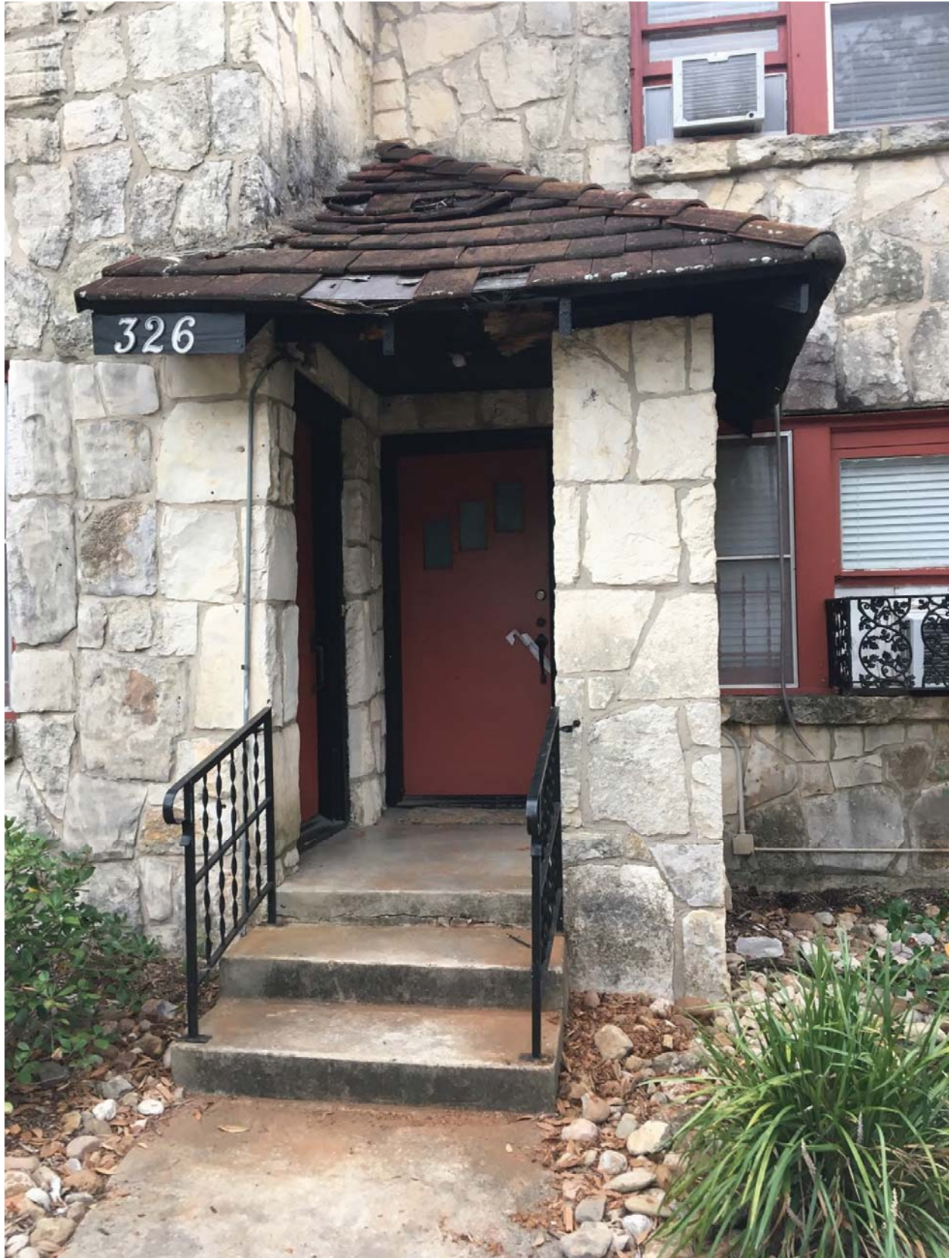
324/326 E. Rosewood Ave. – Front roof in poor condition
