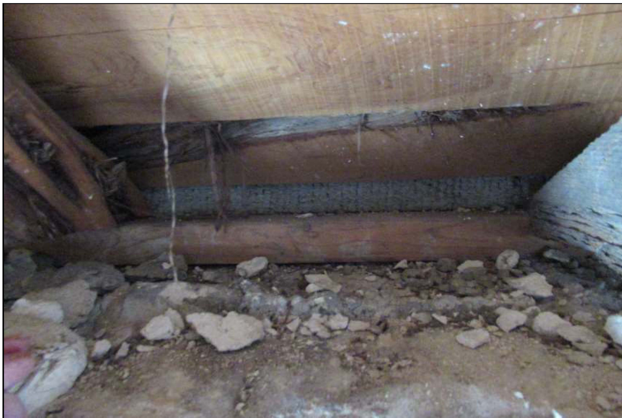
15. View W Top of west wall illustrating concrete beam across the top. Also visible is the lathe and plaster of the front porch stucco.
