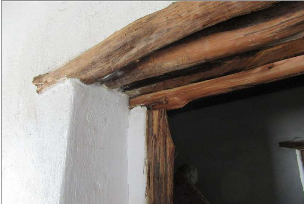
13. View NW Detail of cedar beams and door jamb
