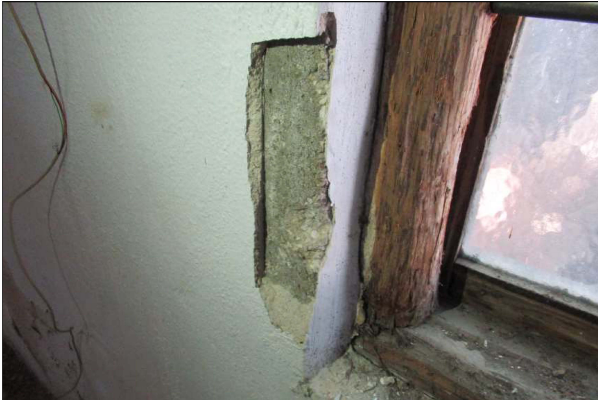
23. View E Poured concrete surround at window jamb
