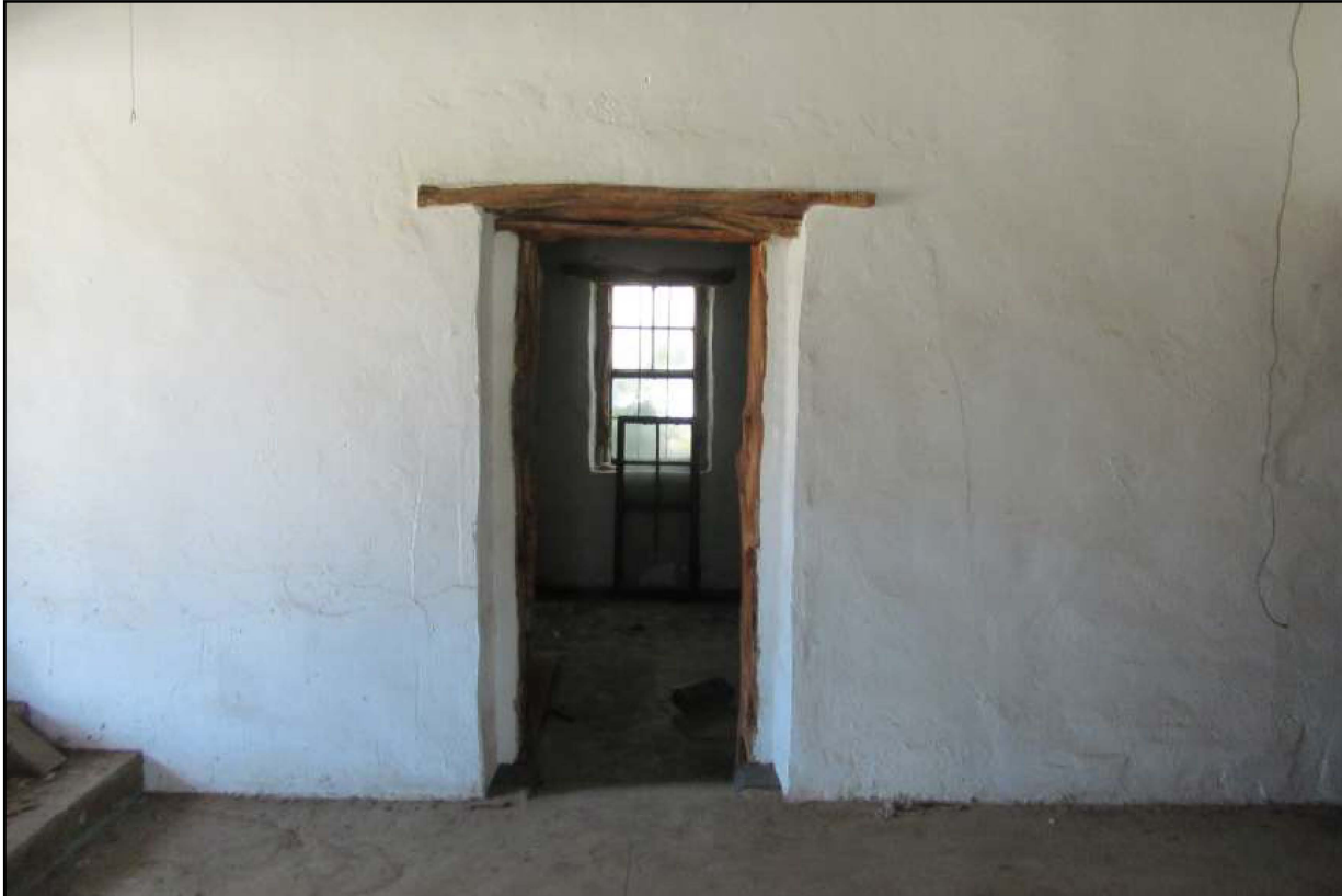
11. View N View of interior wall and door opening with new door frame and header
