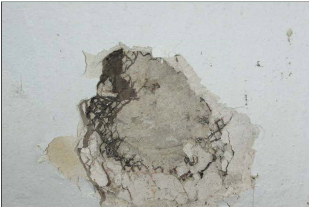
24. View W Exploratory hole with plaster and lathe on caliche wall
