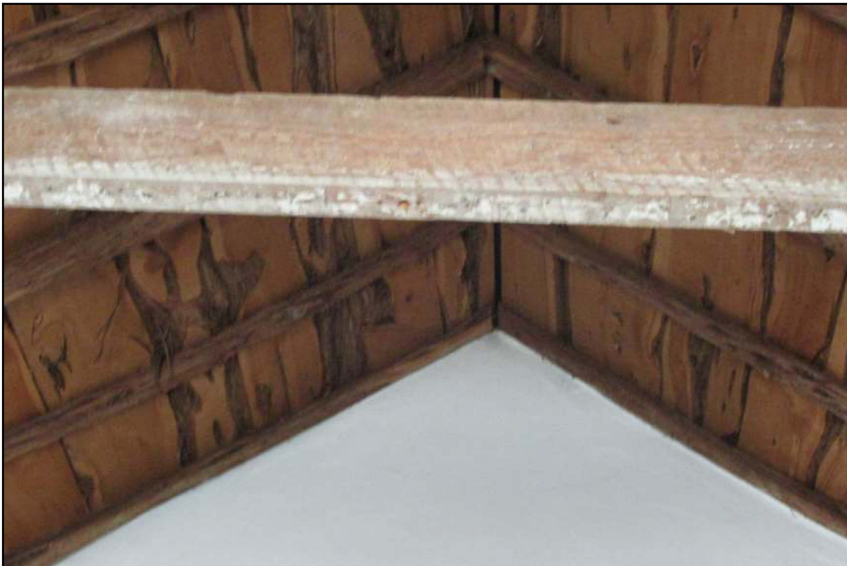
12. View N Ceiling detail at gable showing new cedar joists and cedar plank decking. Recycled wood perlin in foreground.
