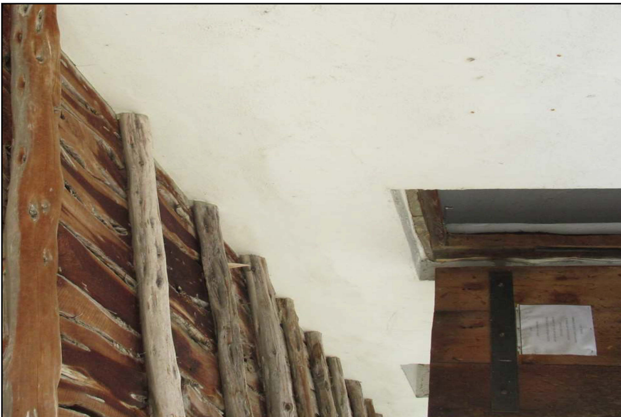
6. View NE Porch roof & door showing new cedar joists and decking, new door and new door frame
