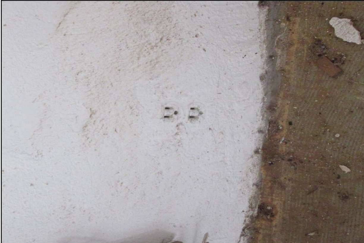
19. Electrical outlet buried in the wall. View E
