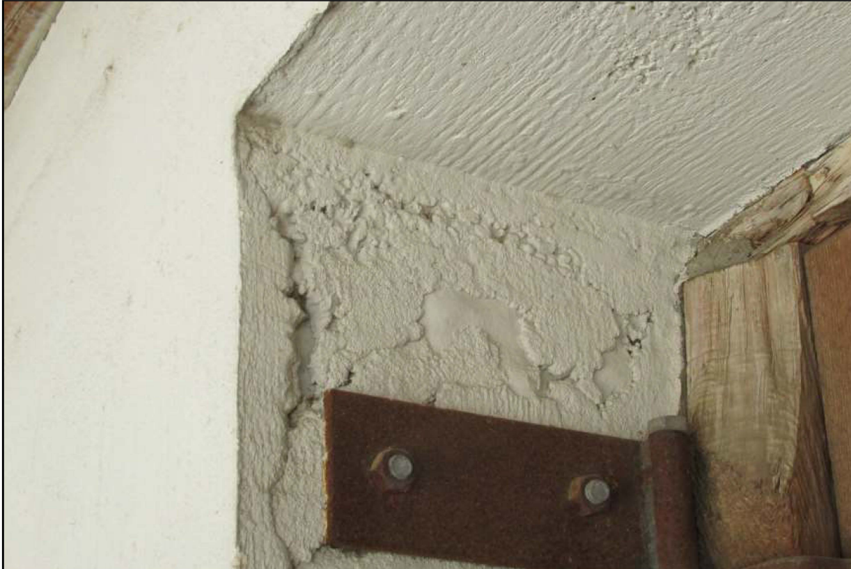
5. View NE Head and jamb of door showing concrete fill
