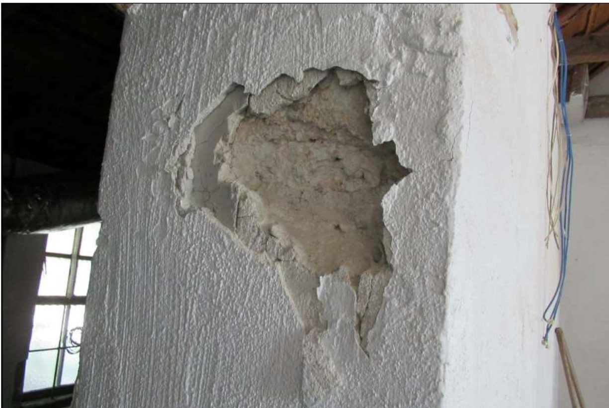
20. View S Detail of expository hole demonstrating layers of plaster and caliche stone wall.
