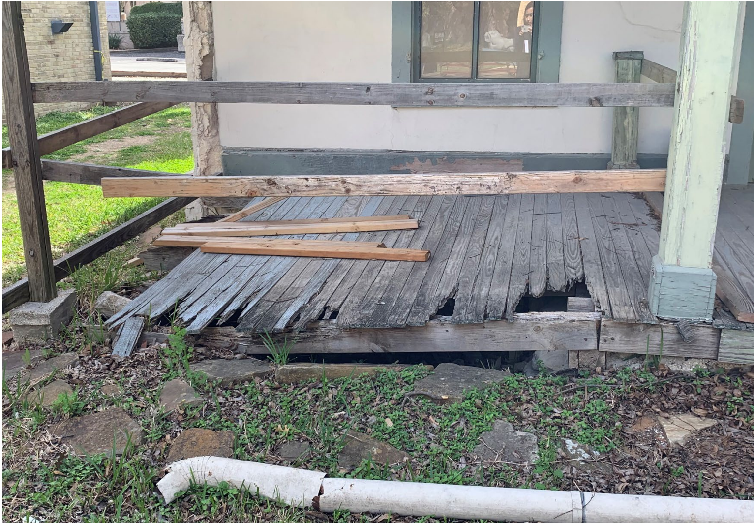
EXISTING NORTH PORCH FRAMING TO BE DEMOLISHED AND RE-BUILT
