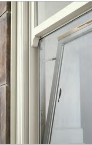
The unobtrusive screen tucks neatly under the checkrail.
