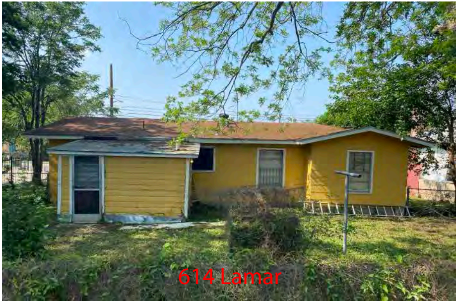
-Horizontal Siding w/8 & 10" Exposure
