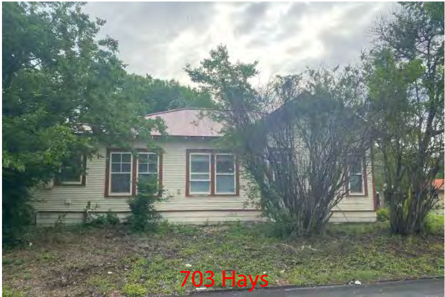
-Horizontal Siding w/4 " Exposure
