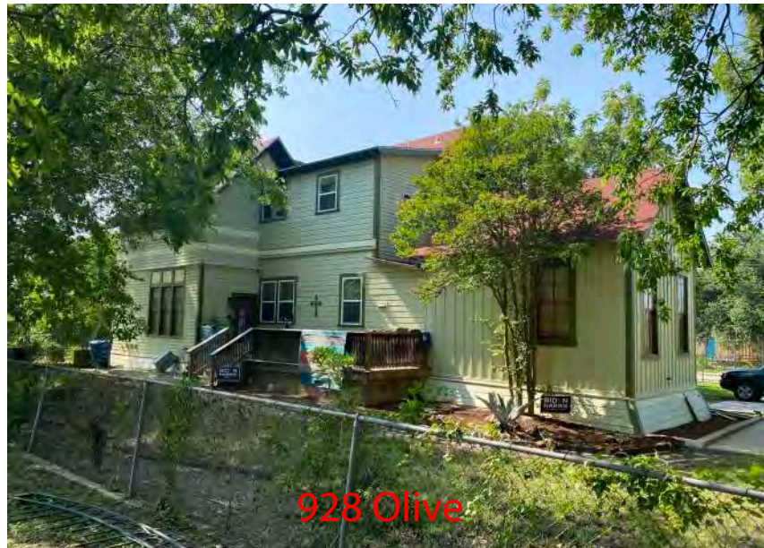
- Vertical 8" Exposure -Horizontal Siding w/6" Exposure
