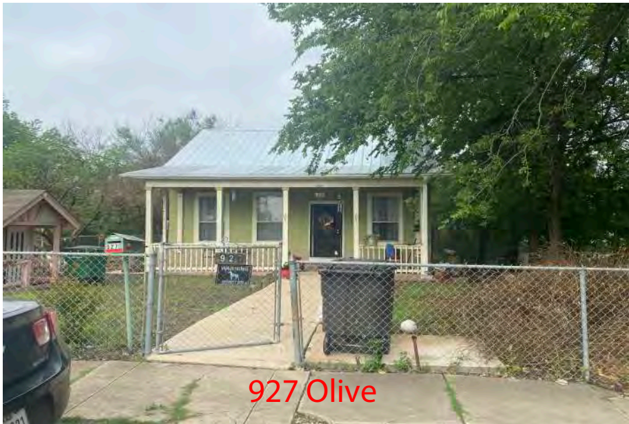
-Horizontal Siding w/8 " Exposure
