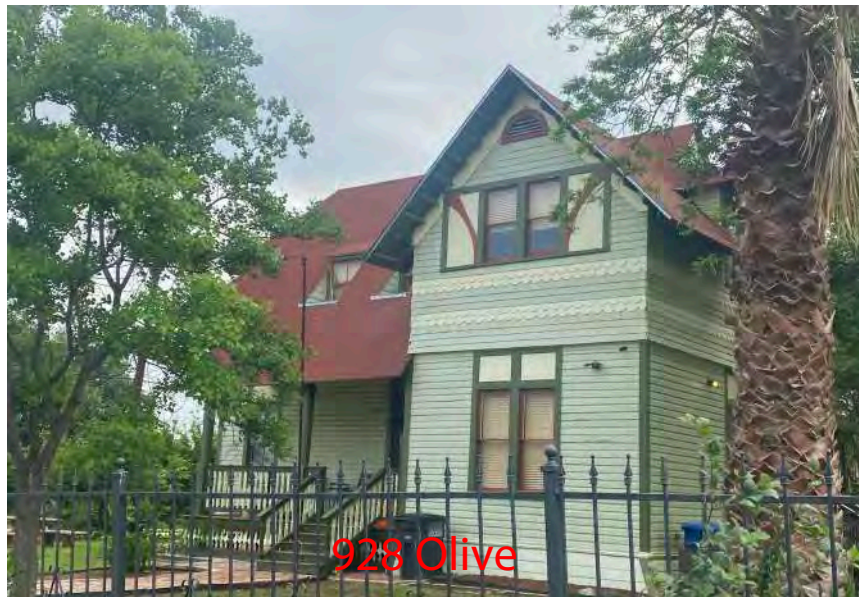
- Horizontal Siding w/4" Exposure -4" Shingles
