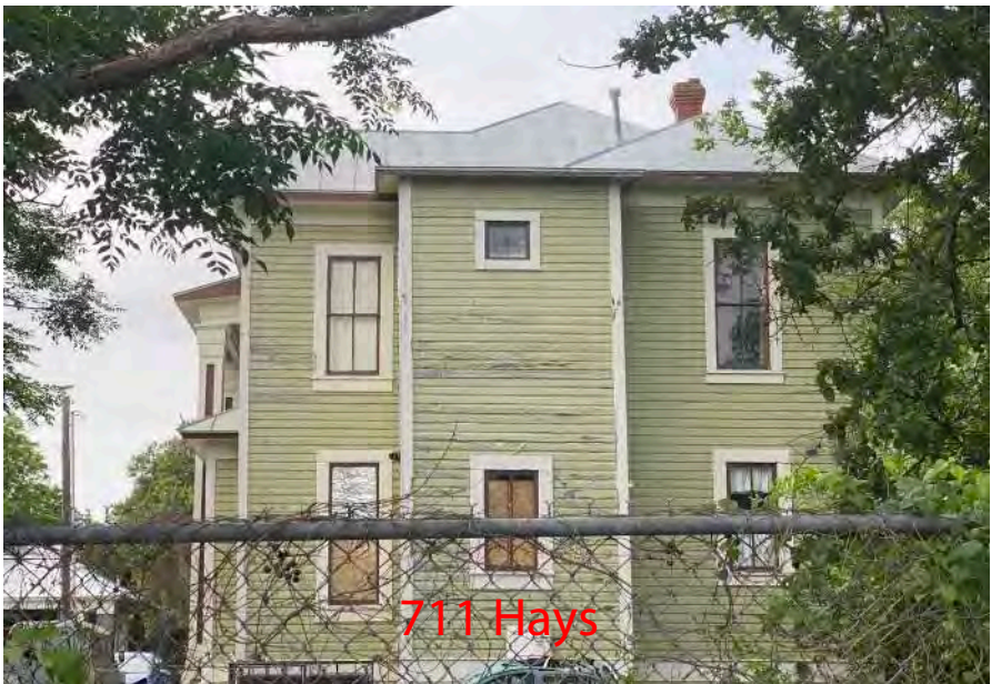
-Horizontal Siding w/4 " Exposure
