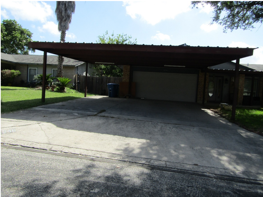
Similar Structure in Area
