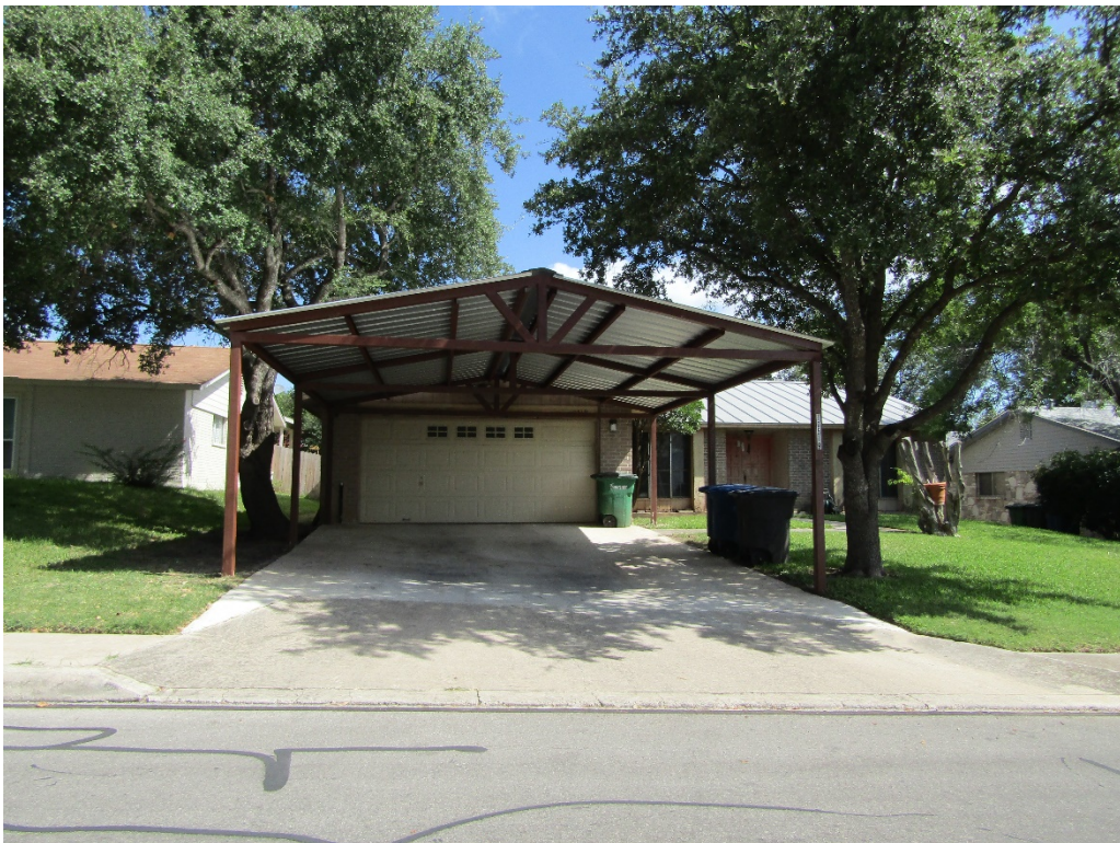
Similar Structure in Area
