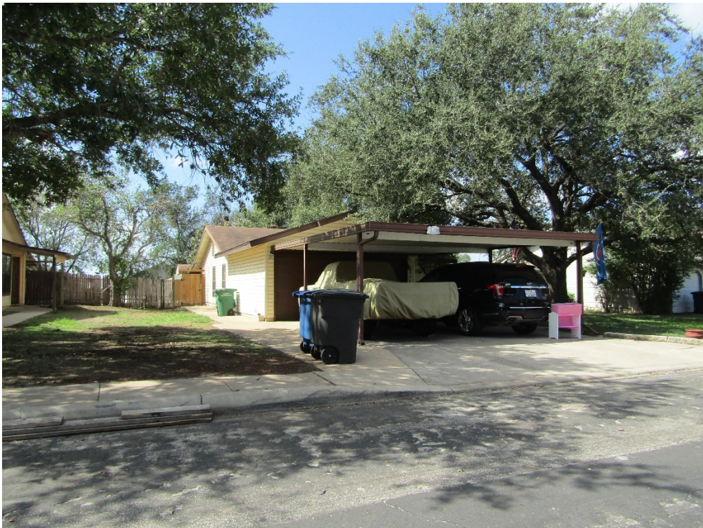
Similar Structure in Area
