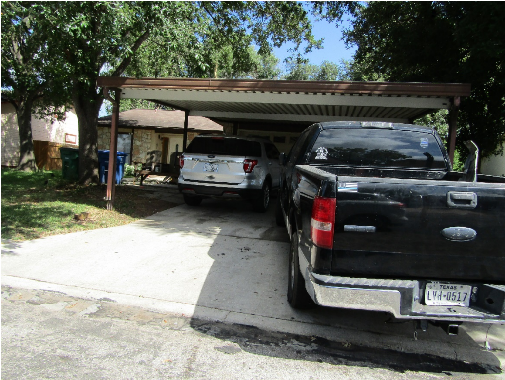
Similar Structure in Area
